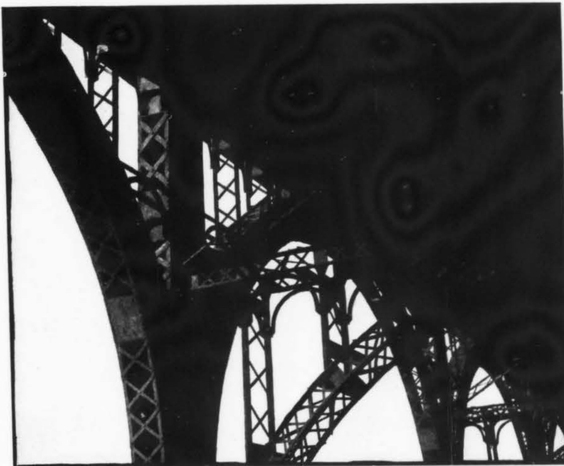
125TH STREET VIADUCT
