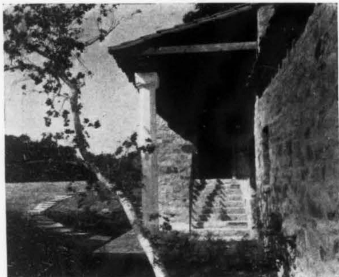
RANCH HOUSE FOR MR. GORDON S. ARMSBY, IN CARMEL VALLEY CLARENCE A. TANTAU, ARCHITECT
