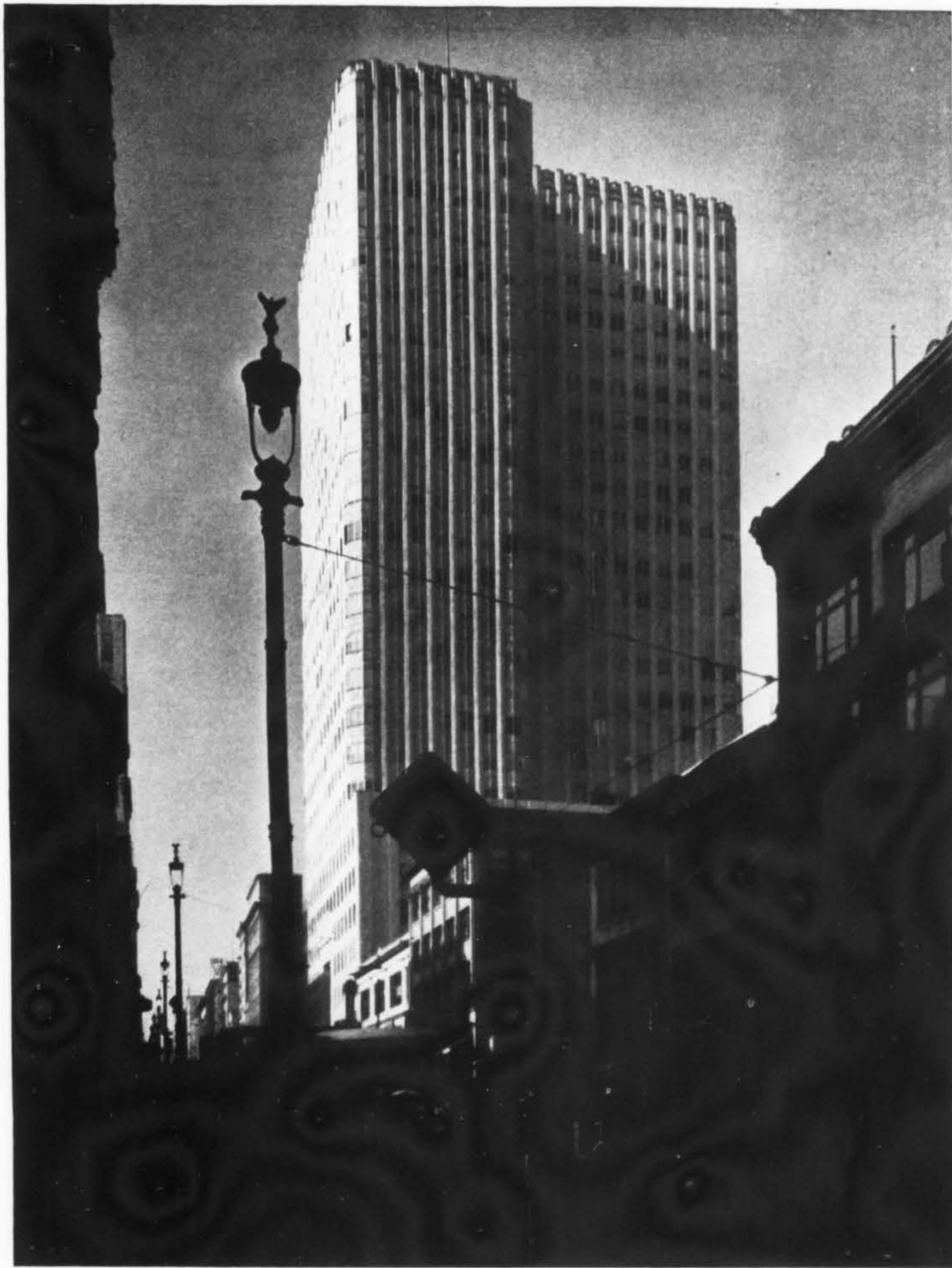
450 SUTTER BUILDING, SAN FRANCISCO
