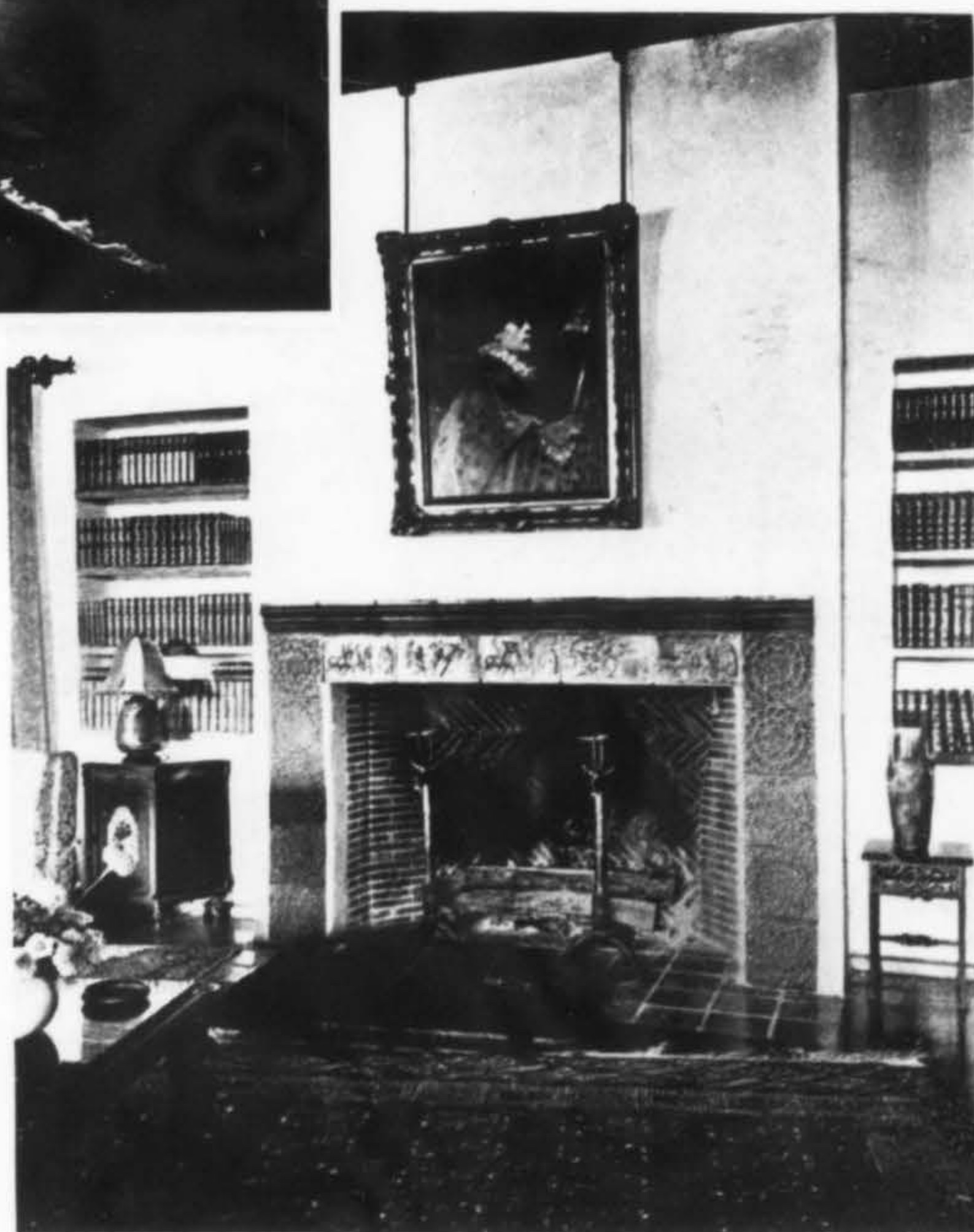
An interesting and unusual tile mantel, lined with Roman brick, is the central feature of the Donaldson living room; above it the chimney breast rises sheer and plain, an excellent background for the fine old painting. No shelf ornaments conflict with this composition, to injure the broadness of scale. Ralph C. Flewelling, A.I.A., Architect.
