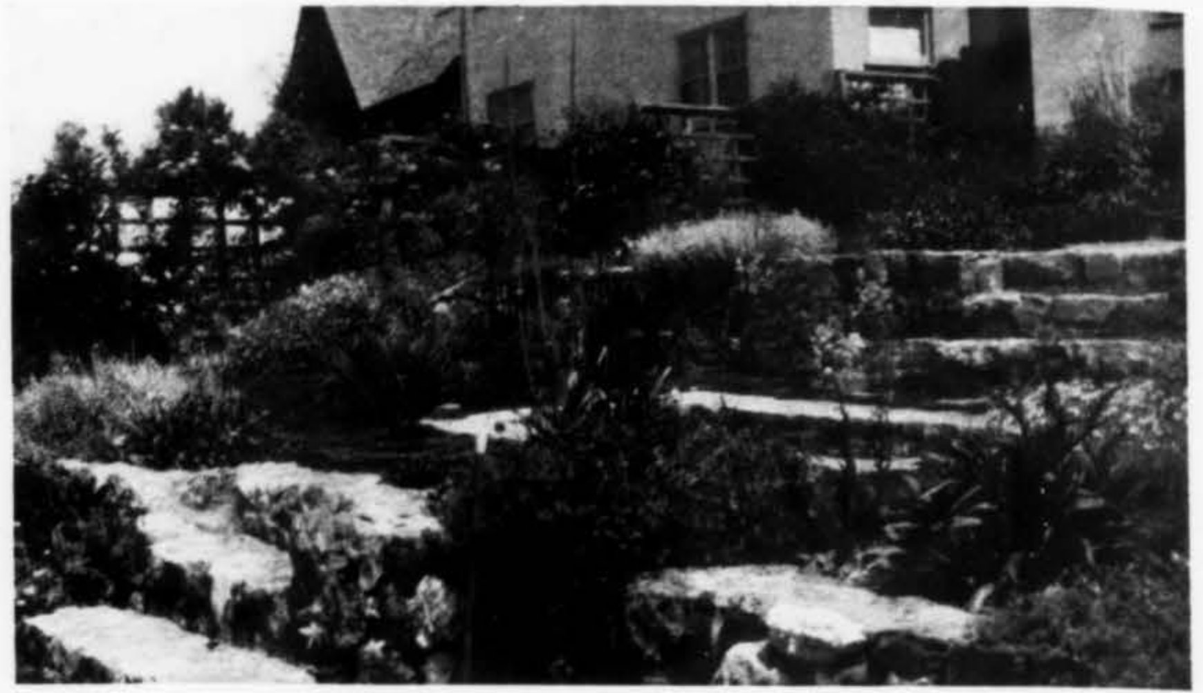
In the terraces of the garden for Professor Geo. D. Louderback in Berkeley, local stone was used for terraces and steps—much better than cement for the effect of rock plants.
