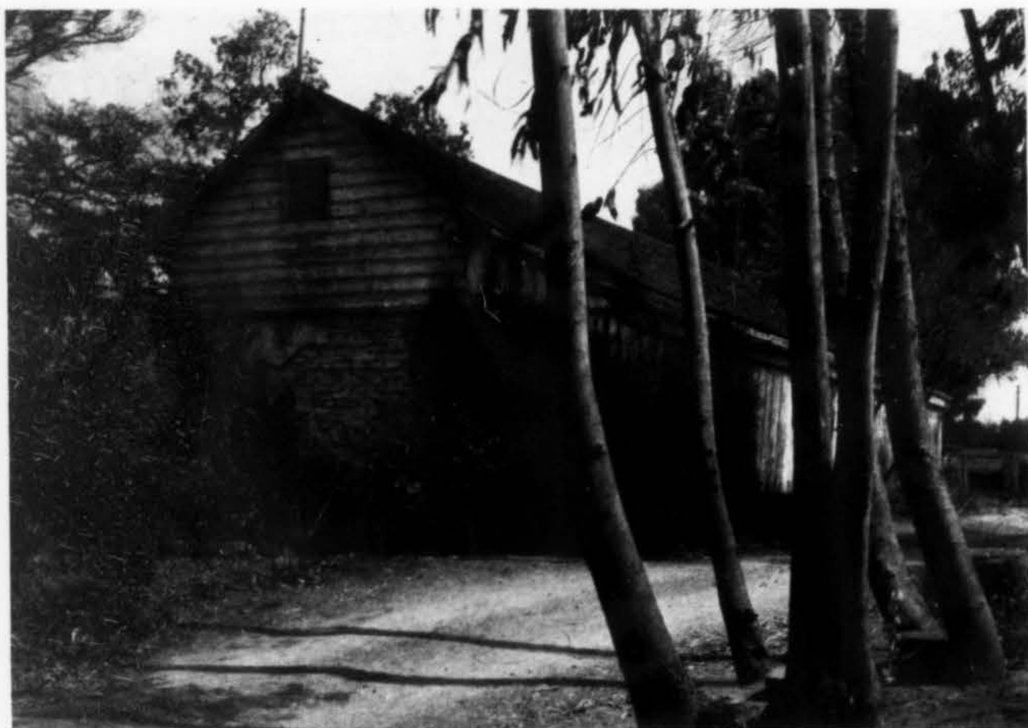
The old barn, showing some of the original hand-made hip tile
