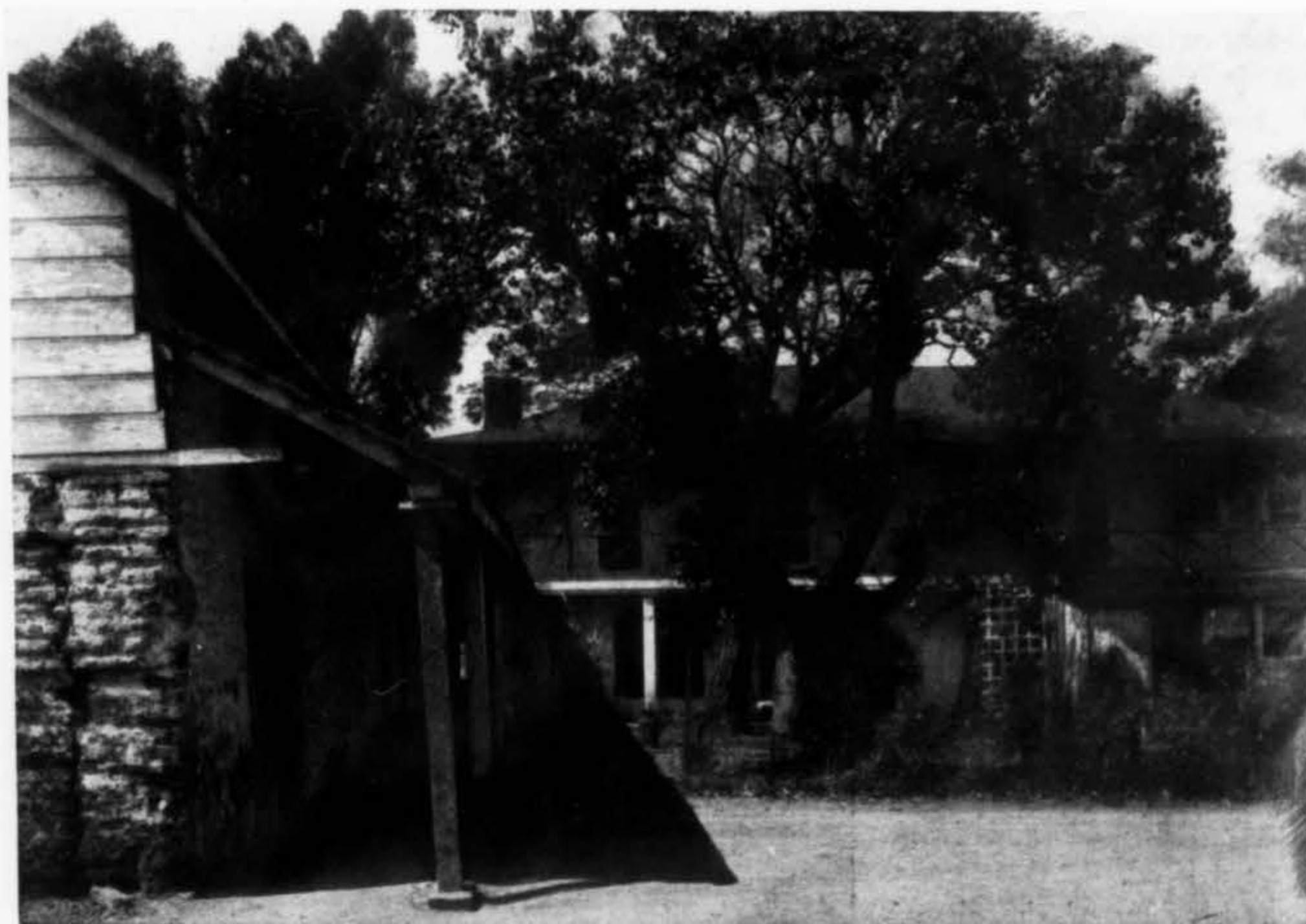
The rear patio from the service wing
