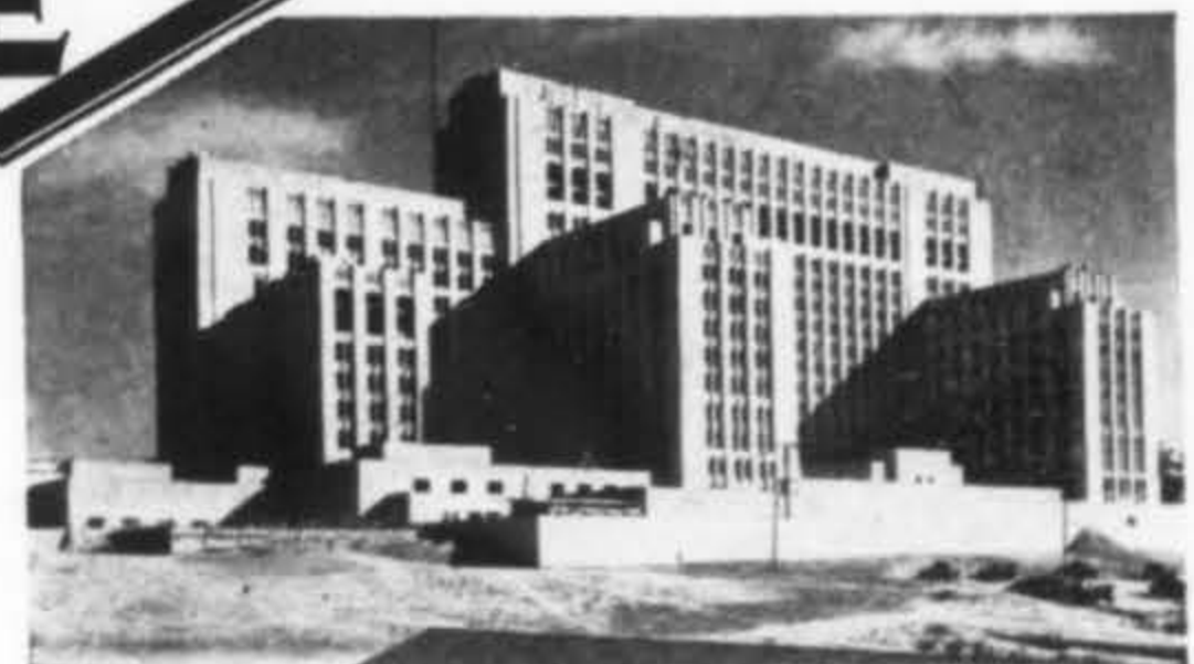
General Hospital now building in Los Angeles to be installed with largest switchboard in the west—Diamond E.
