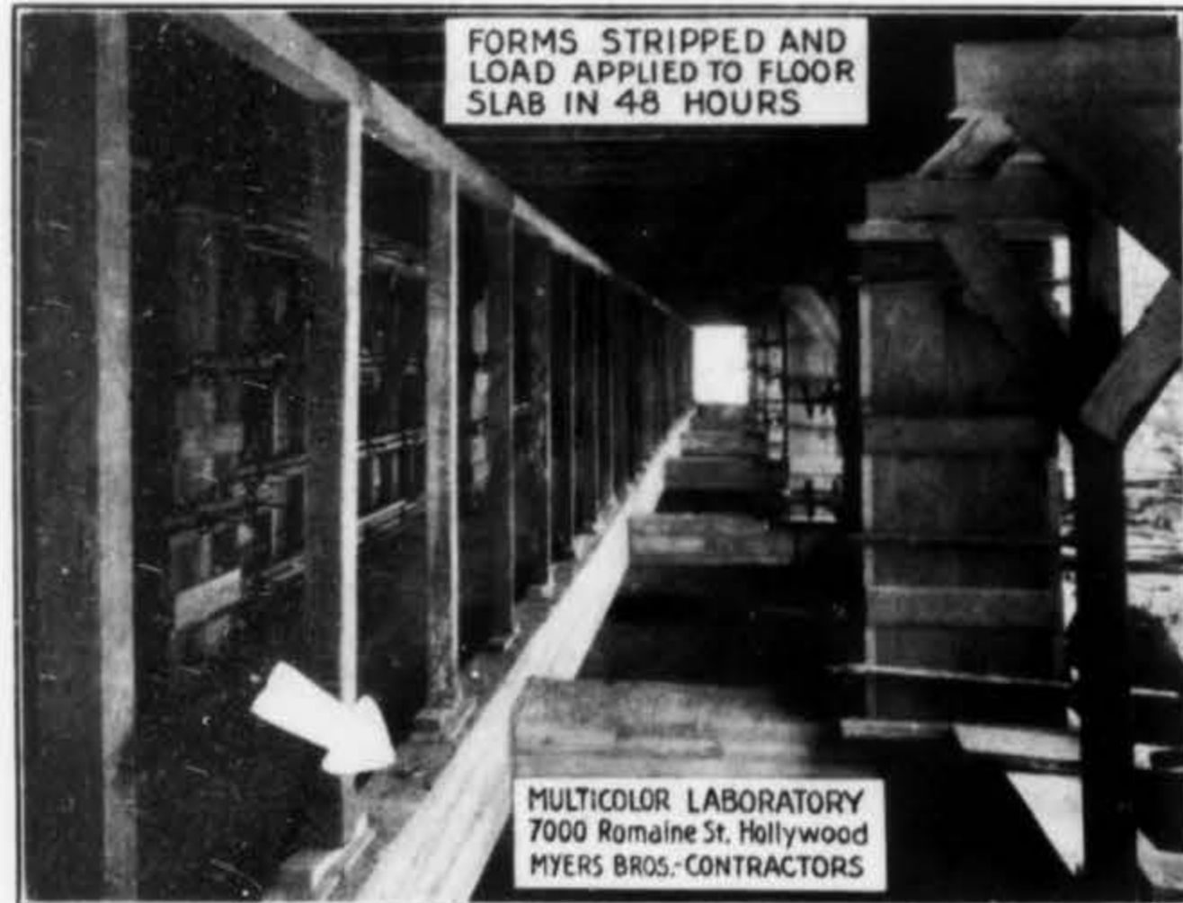
Lower Floor Slab Poured 8/15—Upper Slab Poured 8/18
