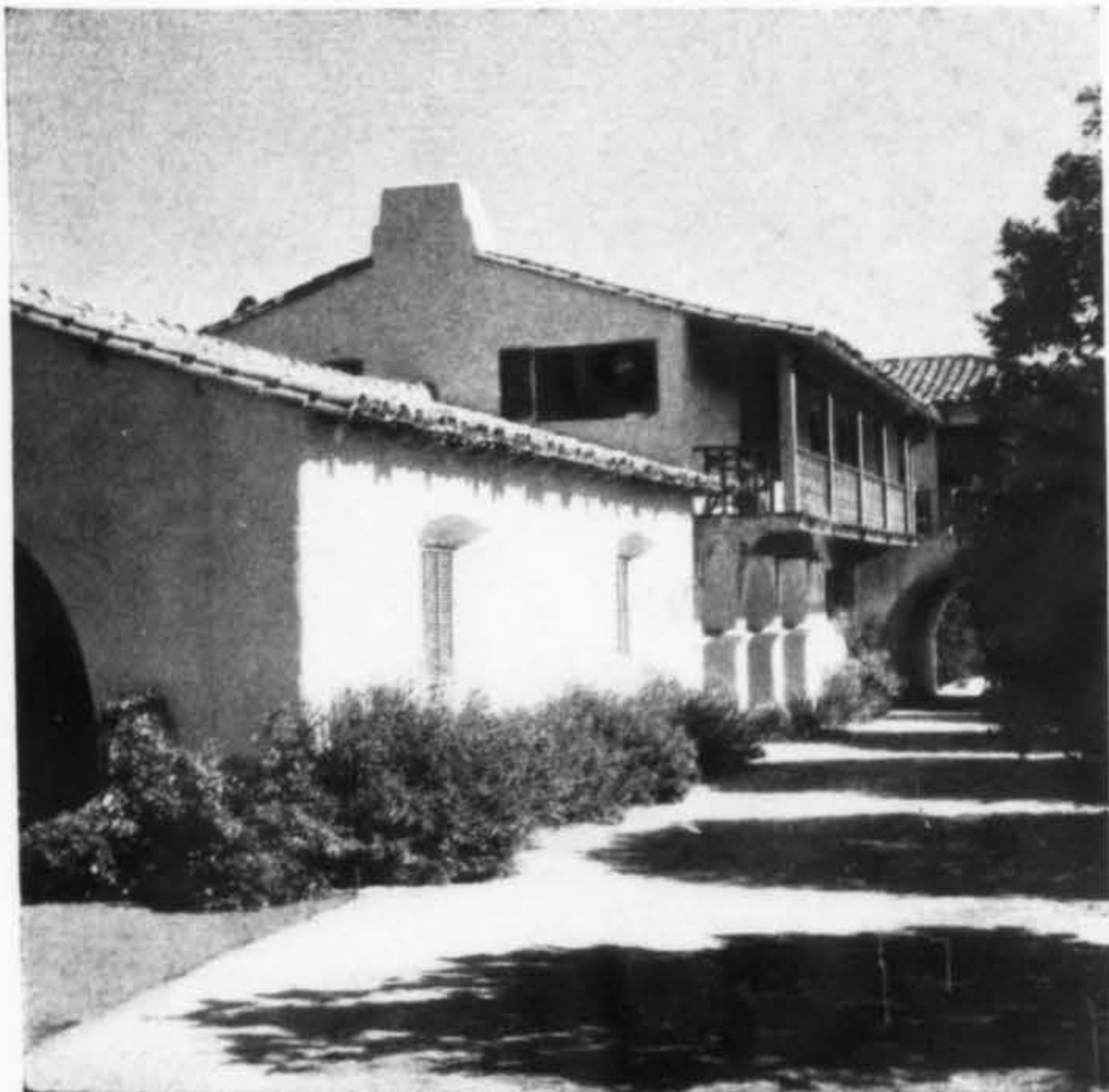
Residence of Mrs. Col. Herman Hall, Sierra Madre; the late Everett Babcock, architect.
