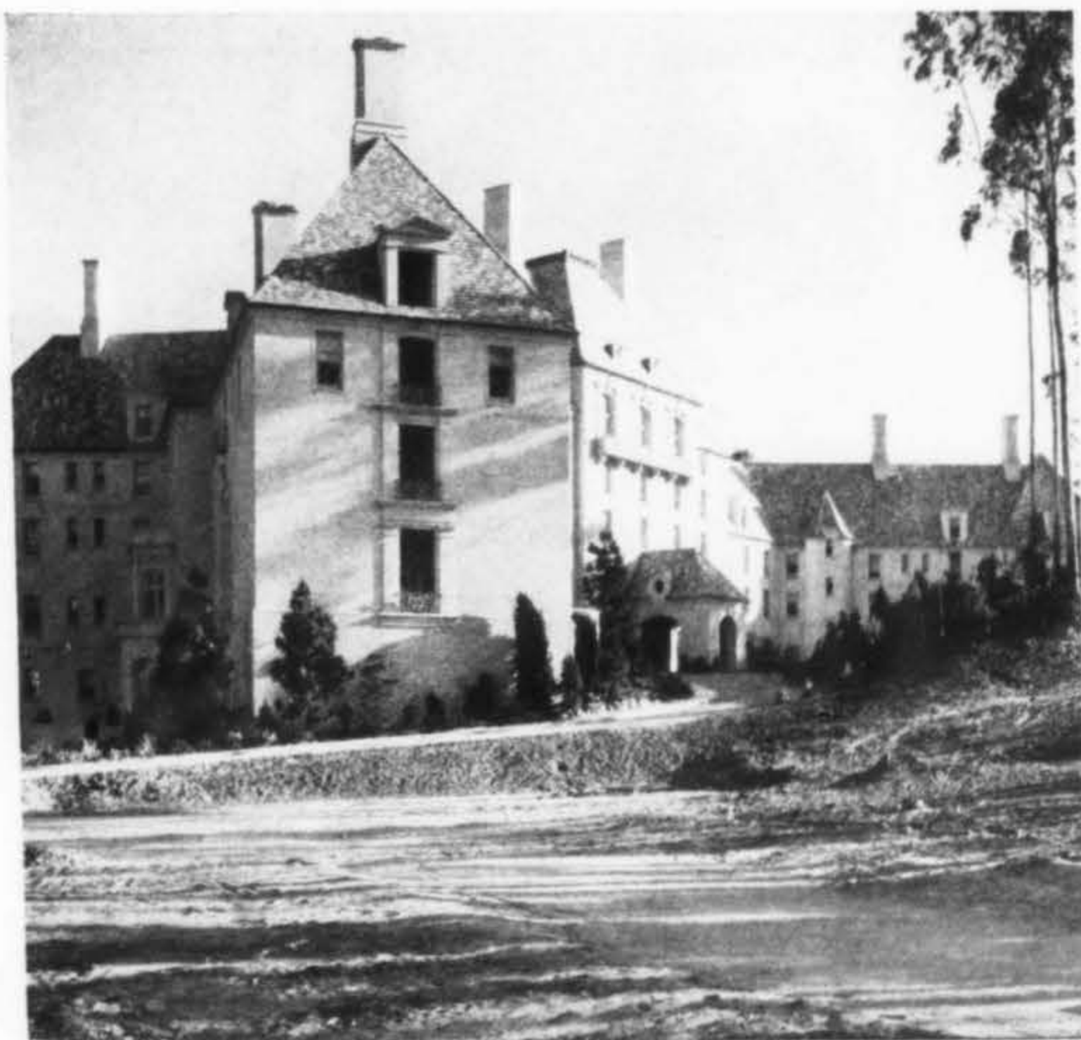
Cleared from the forest for entrance drive and future garden.
