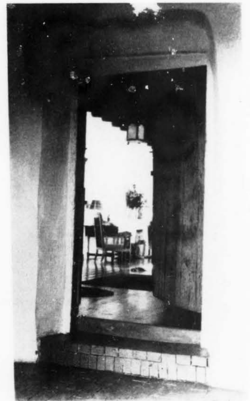
The original arch, lintel and door open into the living room.
