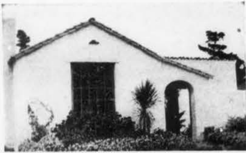
PEBBLE BEACH STUDIO OF DOWSETT-RUHL COMPANY BUILDERS MAIN OFFICE - RUSS BLDG. SAN FRANCISCO
