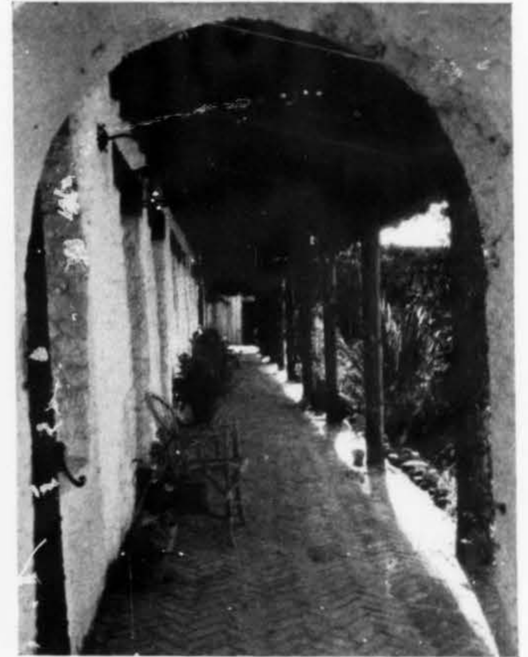
Porch floors in Mr. Mack's hacienda were made of brick laid in "herring-bone" pattern, then scraped to give a natural worn surface.
