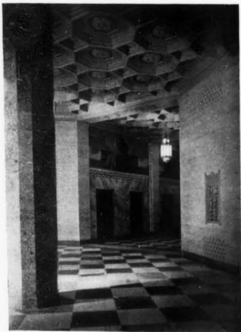
MAIN LOBBY—SOUTHERN CALIFORNIA EDISON BUILDING ALL ORNAMENTAL PLASTERING AND ALL MODELS for MARBLE AND WOOD CARVING
