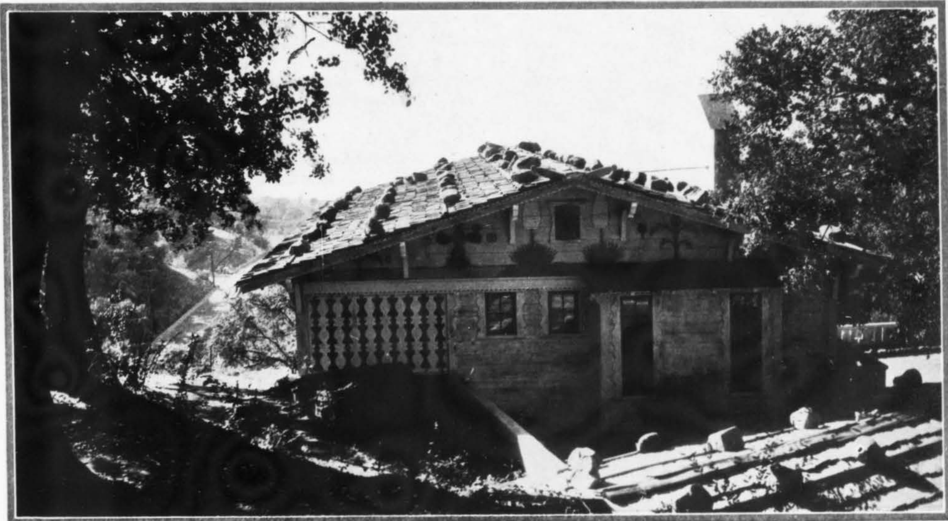
The hill slopes up steeply back from the Guest-house, whose first story is devoted to garage and storage space. In the gable ends are painted decorations of desert plants—prim, and yet gay. In justice to Santa Barbara, we must own that stones are not needed to keep a roof from blowing away.
