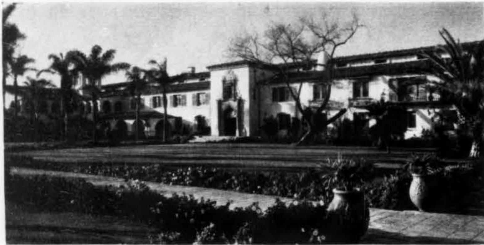
Sisalkraft was used under the stucco on this hotel
