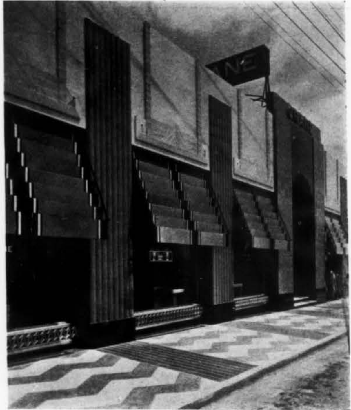
The louver type awning has many advantages. It slides into a pocket at the window head, when not in use. Morgan, Walls & Clements, architects.
