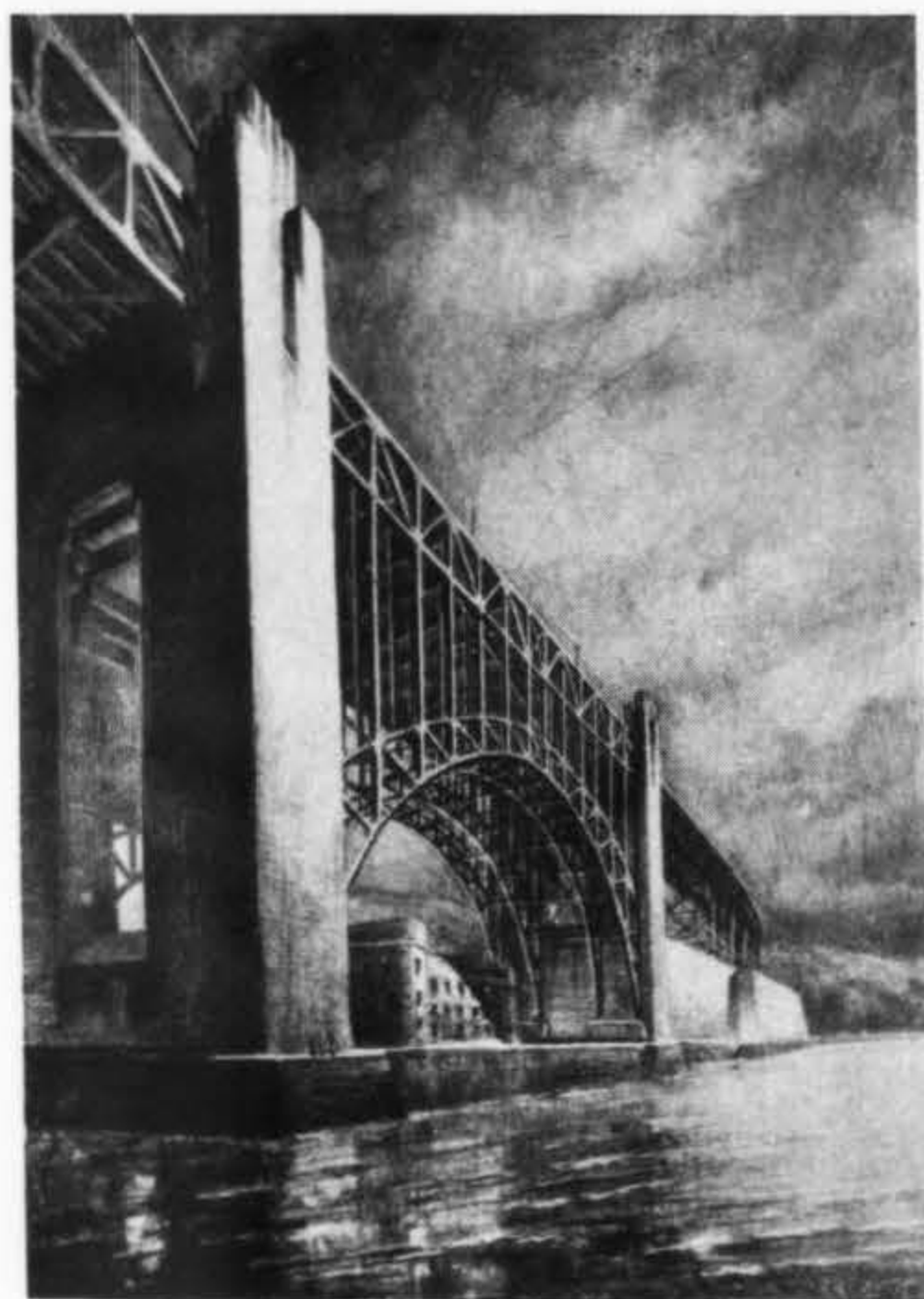
Approach to the bridge from San Francisco; old Fort Point remains undisturbed, under the arch of the great steel trusses.
