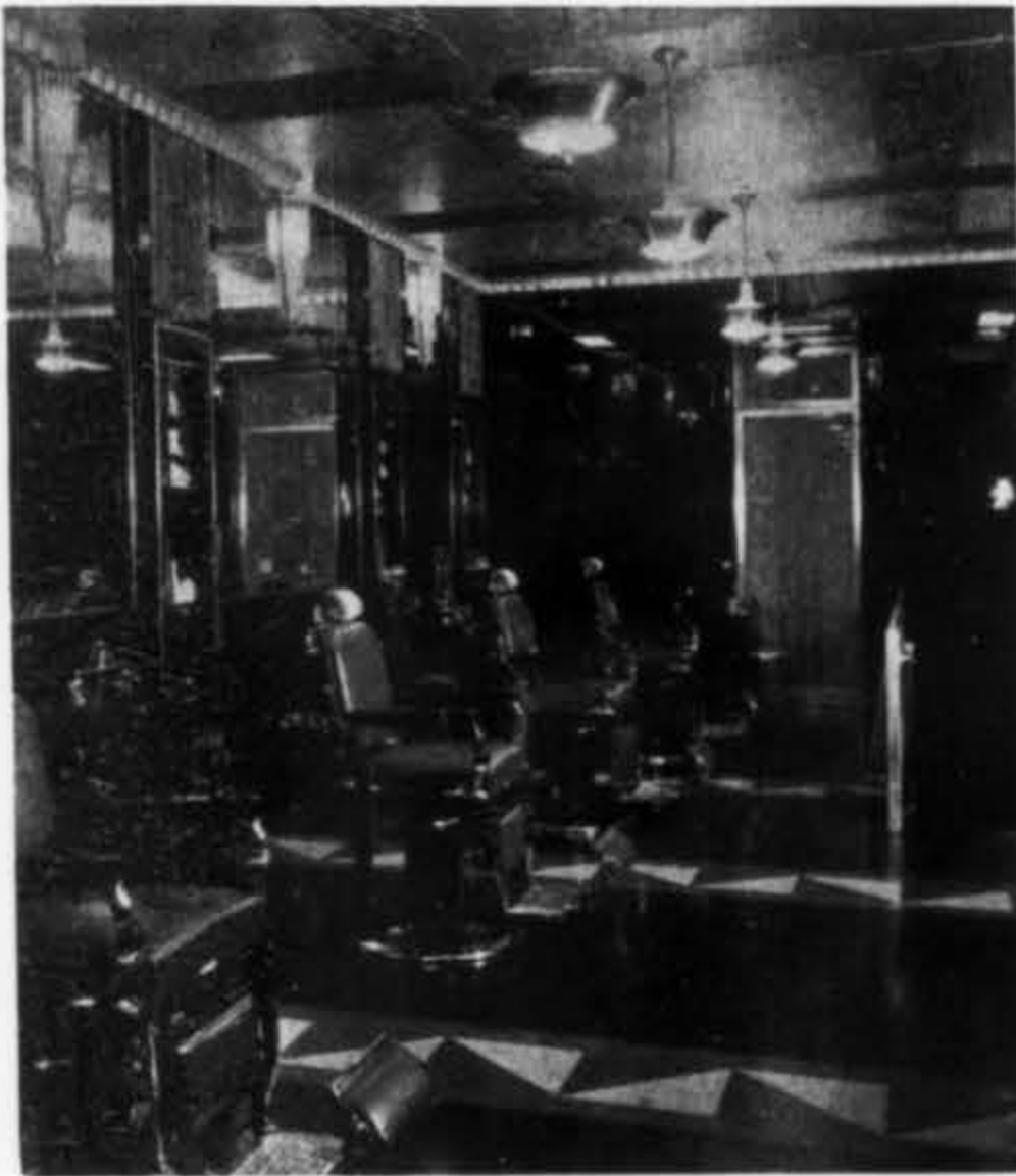
This barber shop has walls of glass, ceiling of metal leaf; grilles are of cast iron, silvered; the floor is rubber tile. Morgan, Walls & Clements, architects.
