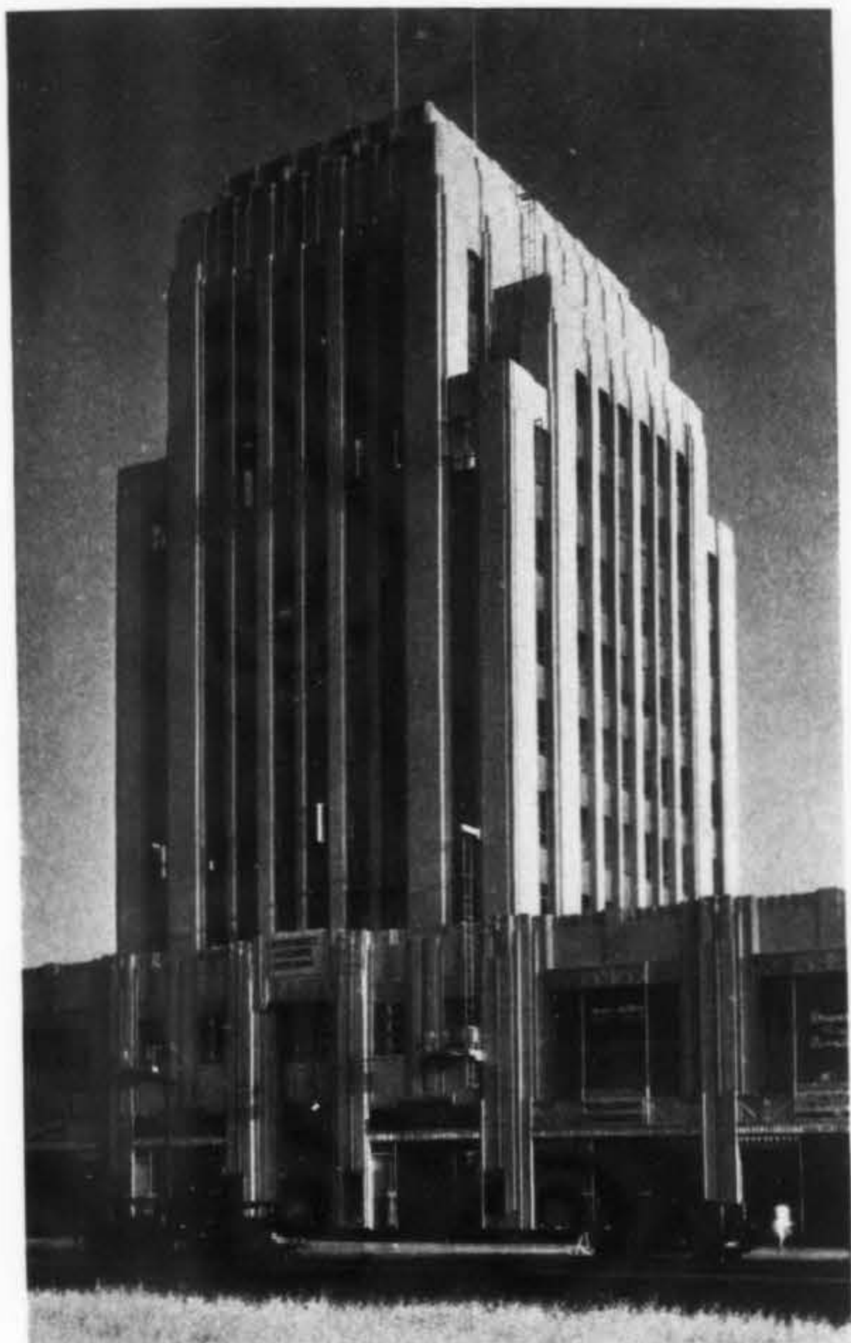
For second story shops, the show windows are here lowered several feet below the floor line for easy visibility from passing automobiles. Below the sign space is a covered awning box. There is a feeling of architectural unity that many modern buildings lack. Morgan, Walls & Clements, architects.
