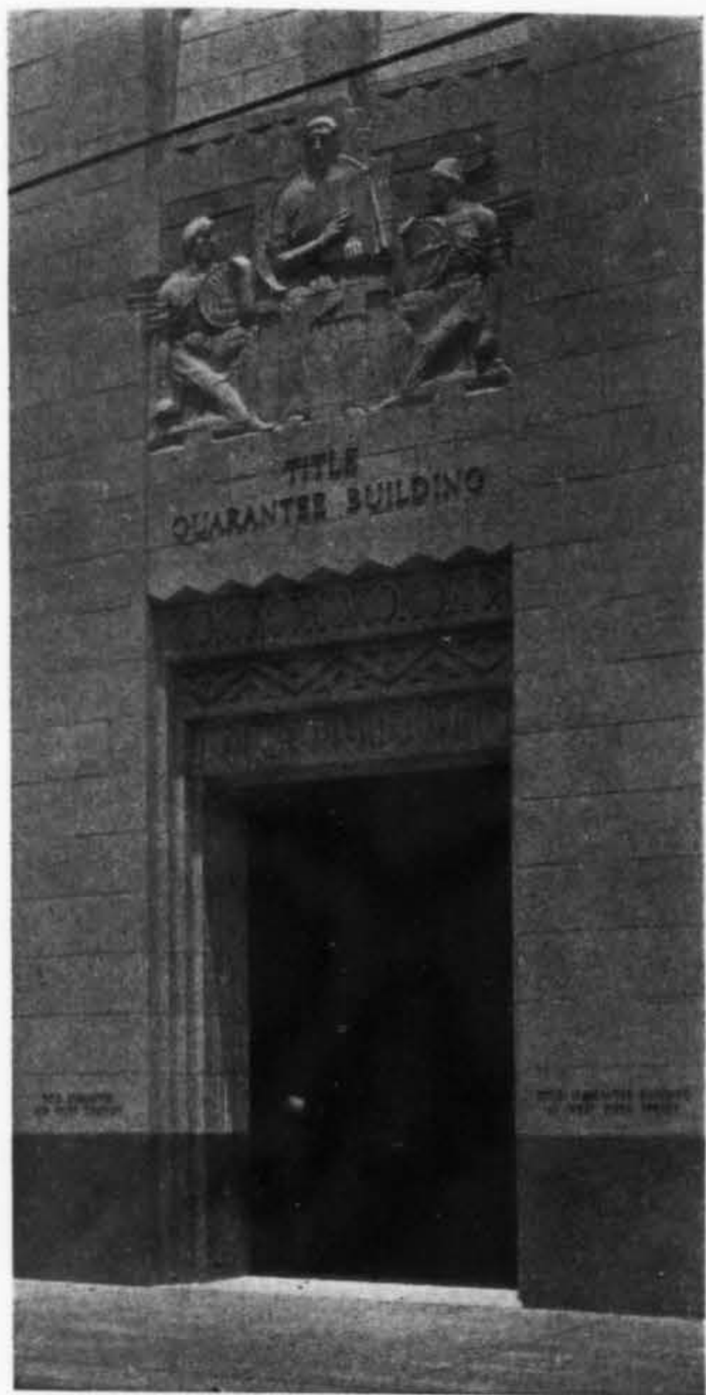
The versatility of terra cotta is well shown in the entrance detail of the Title Guarantee building; from granite base up, the entire facade is faced with baked clay, including the overdoor sculpture in high relief. Eugene Maier-Krieg, sculptor; John Parkinson and Donald B. Parkinson, architects.
