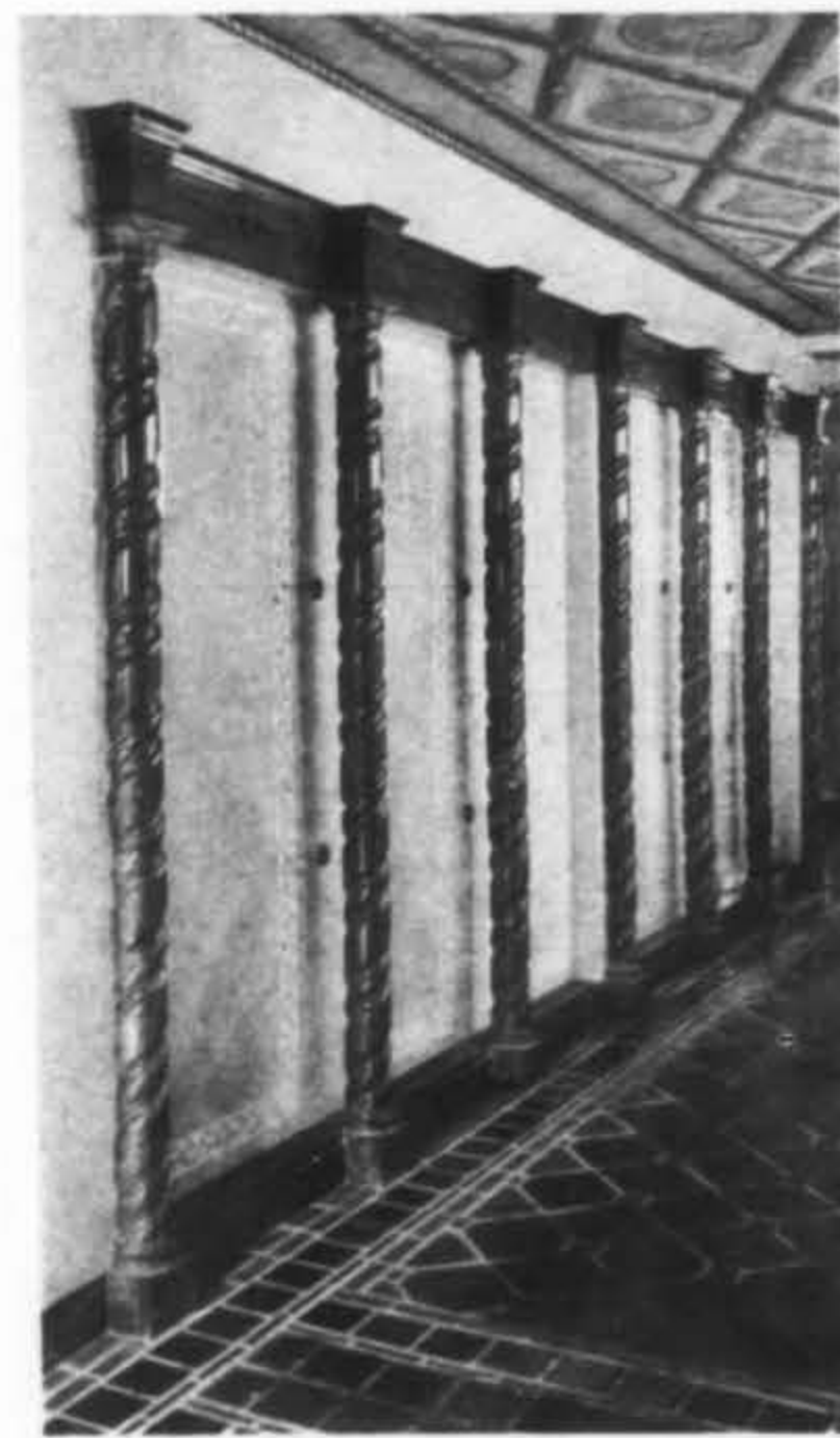
Above,—fancy columns turned with special machinery, for a mausoleum.
