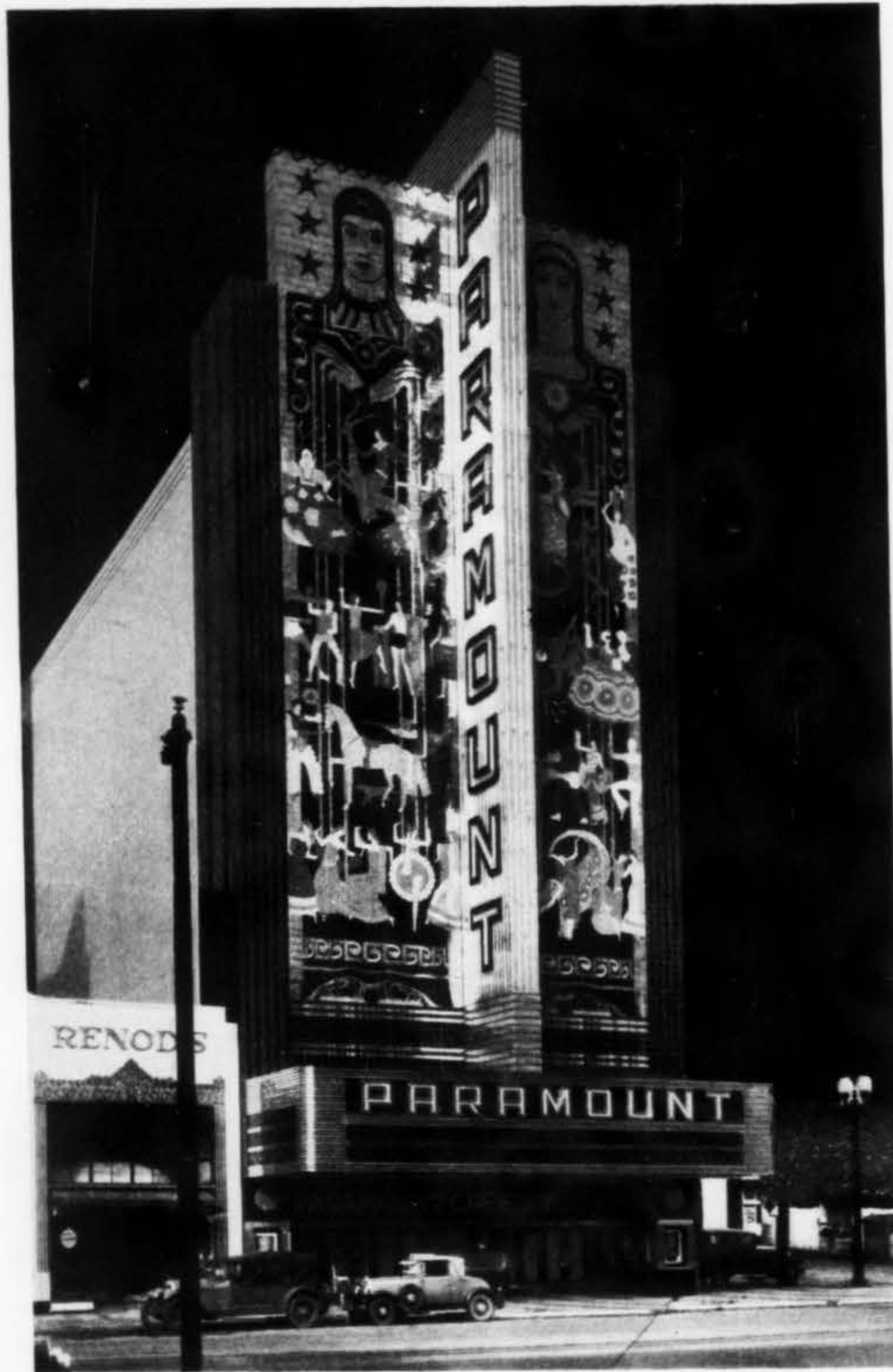
THE PARAMOUNT THEATRE—OAKLAND, CALIFORNIA ARCHITECTS, MILLER & PFLUEGER GENERAL CONTRACTOR, GEORGE WAGNER
