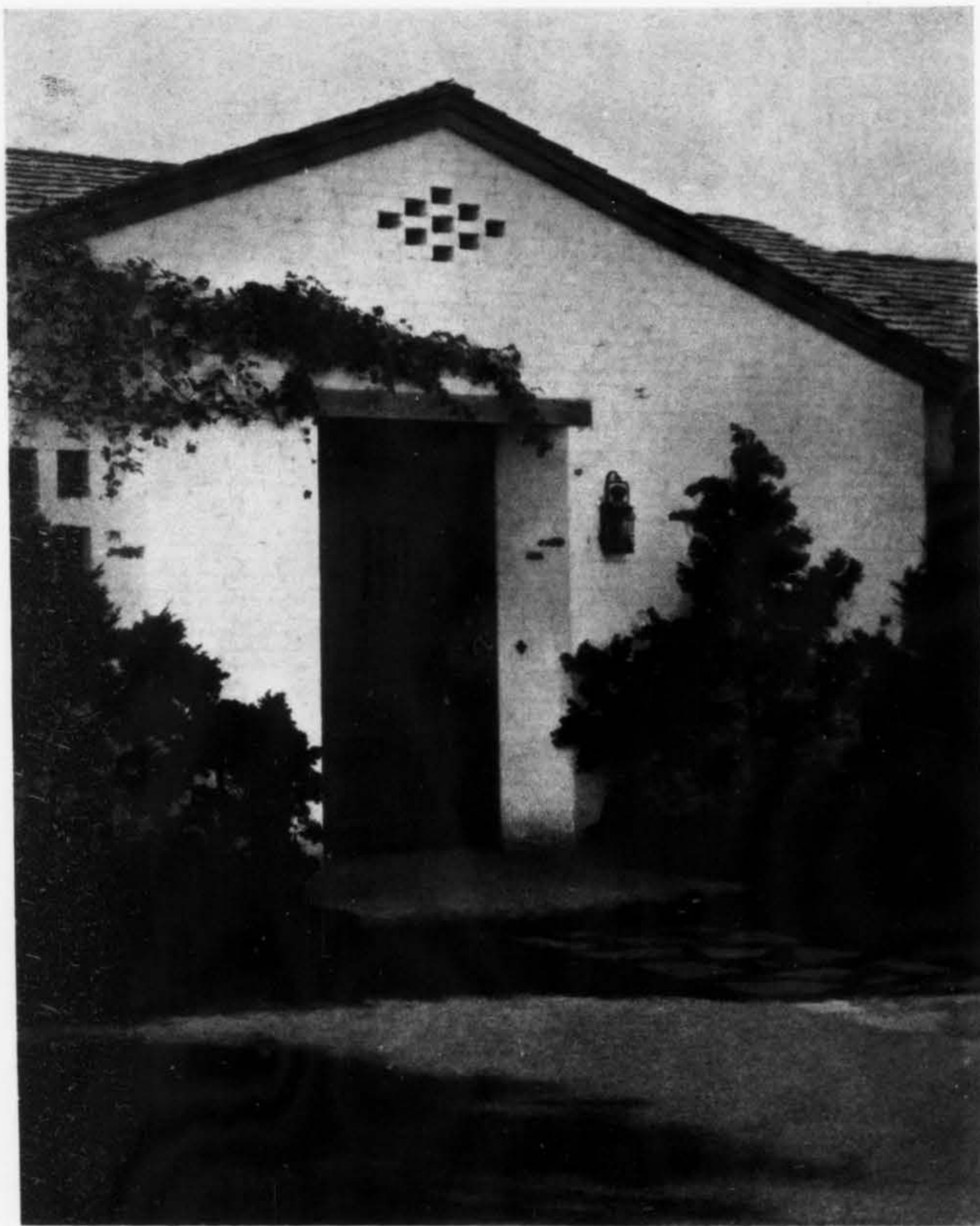
The entrance gable to Mr. Curtis Cate's home in Carpinteria has the charm that endures, because of simplicity and good proportions. Reginald D. Johnson, F. A. I. A., was the architect.
