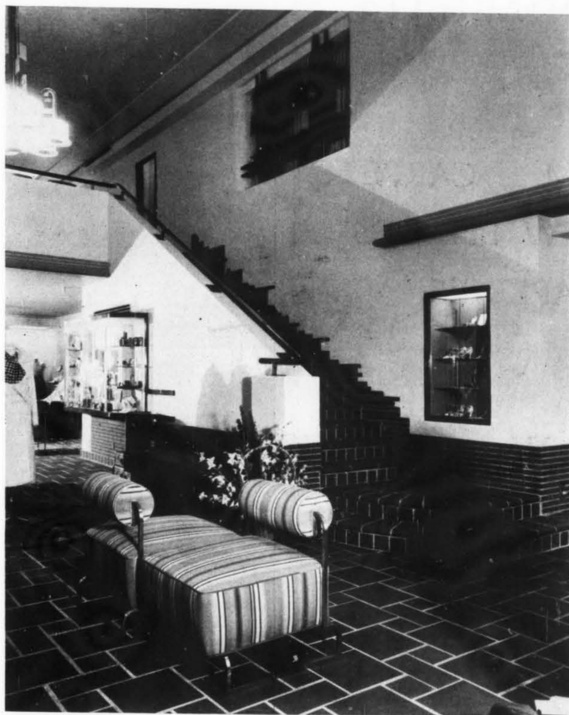
A novel and interesting use of Lincoln Quarry Tile on the floor and wainscot of Bullock's new store in Westwood Village, Los Angeles—John and Donald B. Parkinson, Architects.
