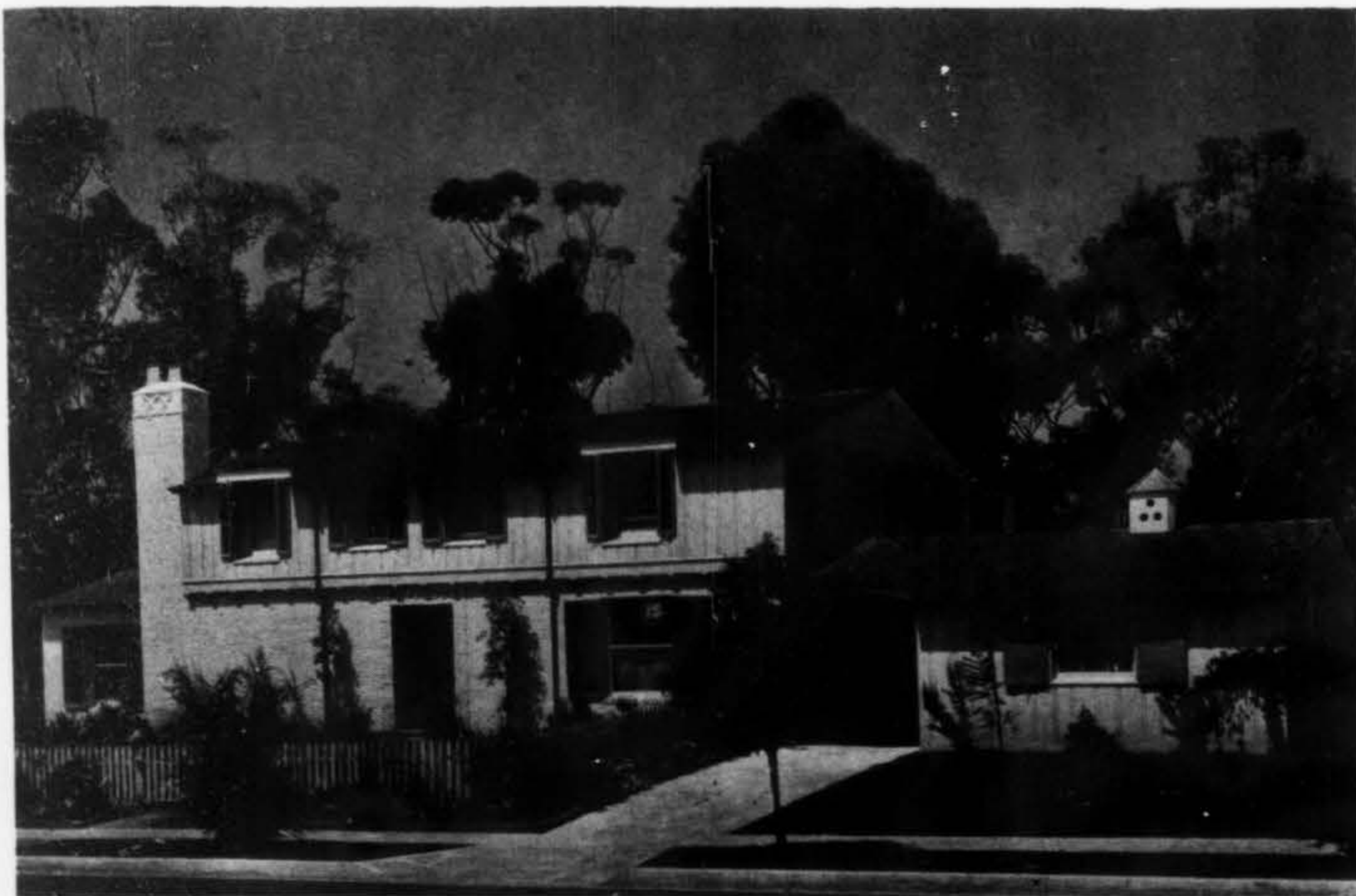
Residence of Mr. and Mrs. W. H. Theobald, Pacific Palisades. Paul R. Williams, architect.
