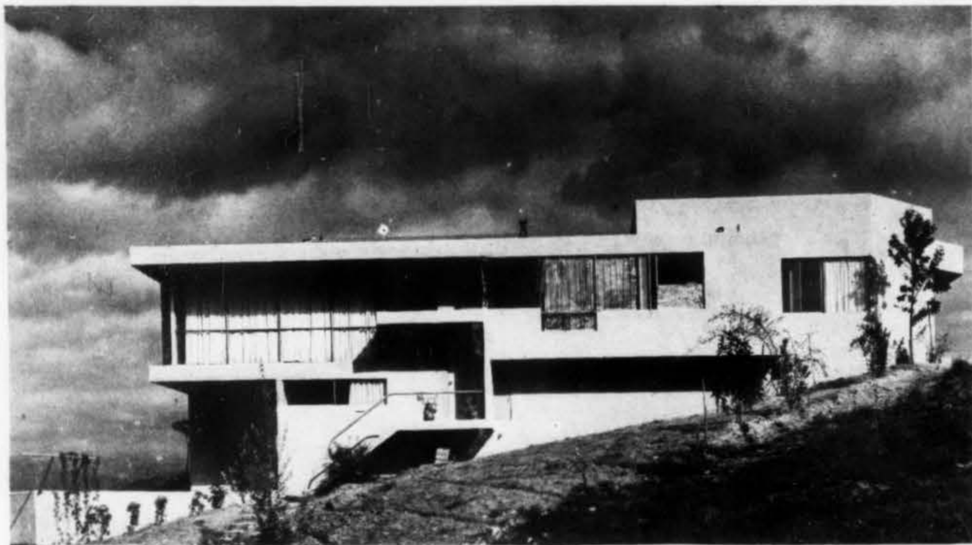
RESIDENCE OF MR. AND MRS. W. OLIVER, LOS ANGELES, CALIFORNIA. R. M. SCHINDLER, ARCHITECT
