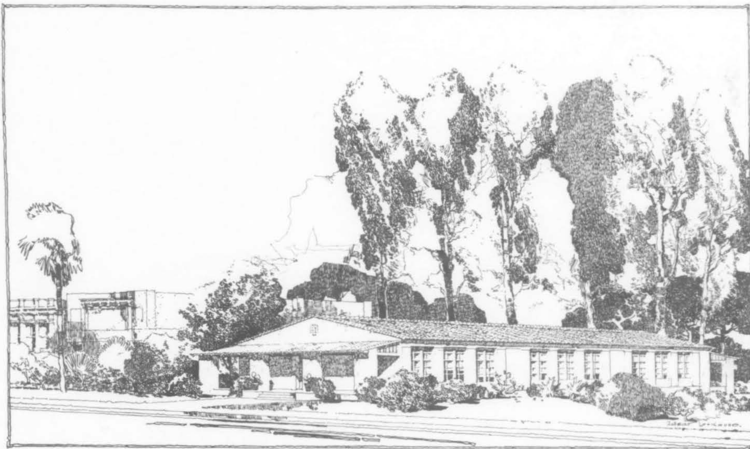
Included in the present Los Angeles school building program is this new eight unit addition to the Lankershim Elementary School. Of early California style, it is to be built of earthquake resistant wood frame with cement Gunitex exterior and metal lath and plaster interior. Henry C. Newton, A.I.A. and Robert D. Murray, A.I.A., architects.
