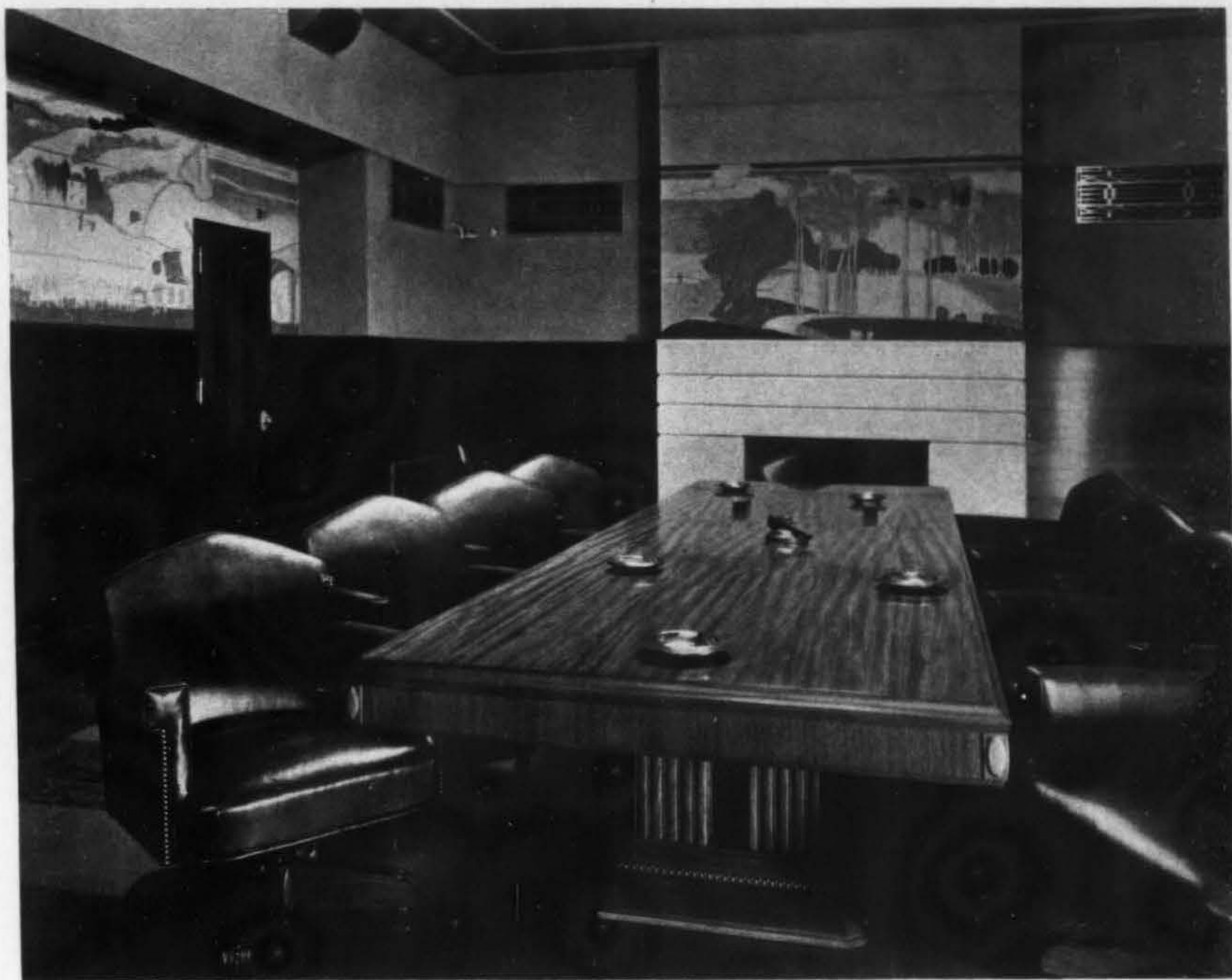
The main banking room is modern and especially pleasing. The walls are acoustic plaster tinted and decorated in water color. The floor is covered with sheet rubber in varying shades. The telephone switchboard at the information desk is housed in an ornamental aluminum cover. By emphasizing the longitudinal lines a feeling of greater depth is secured.
