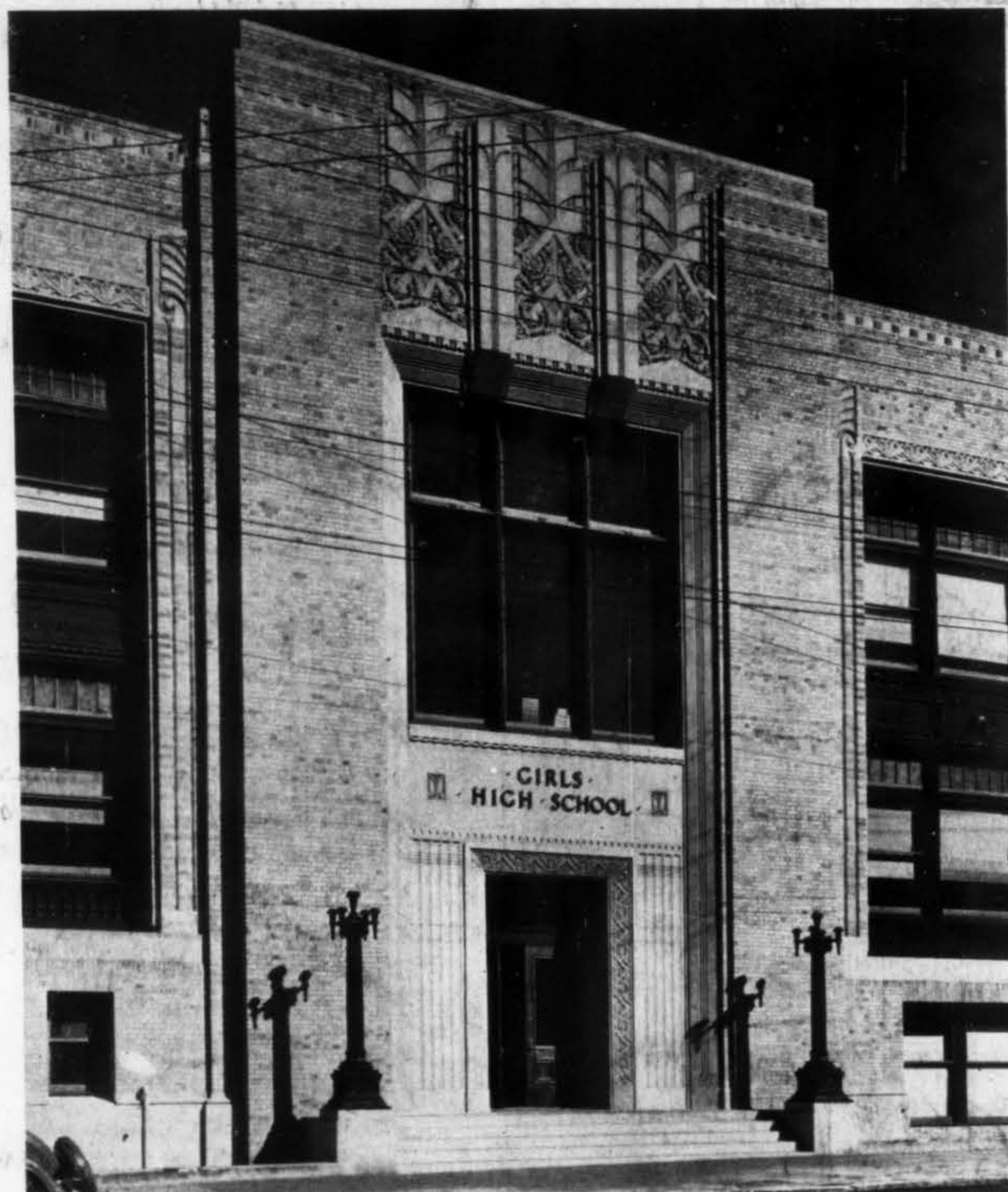
Main Entrance, Girls' High School, San Francisco
