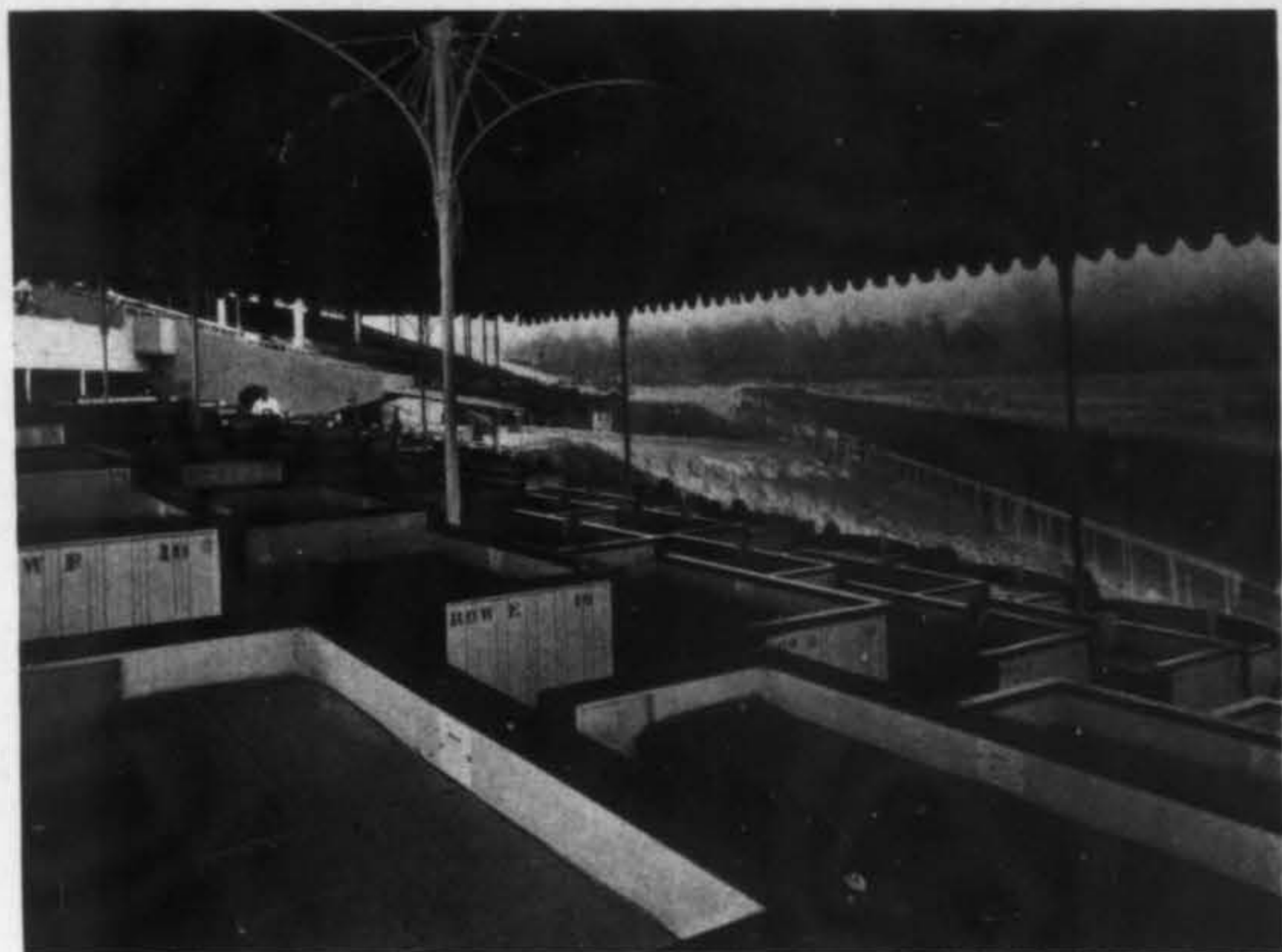
View from the new clubhouse addition showing grandstand and new bleachers in distance.
