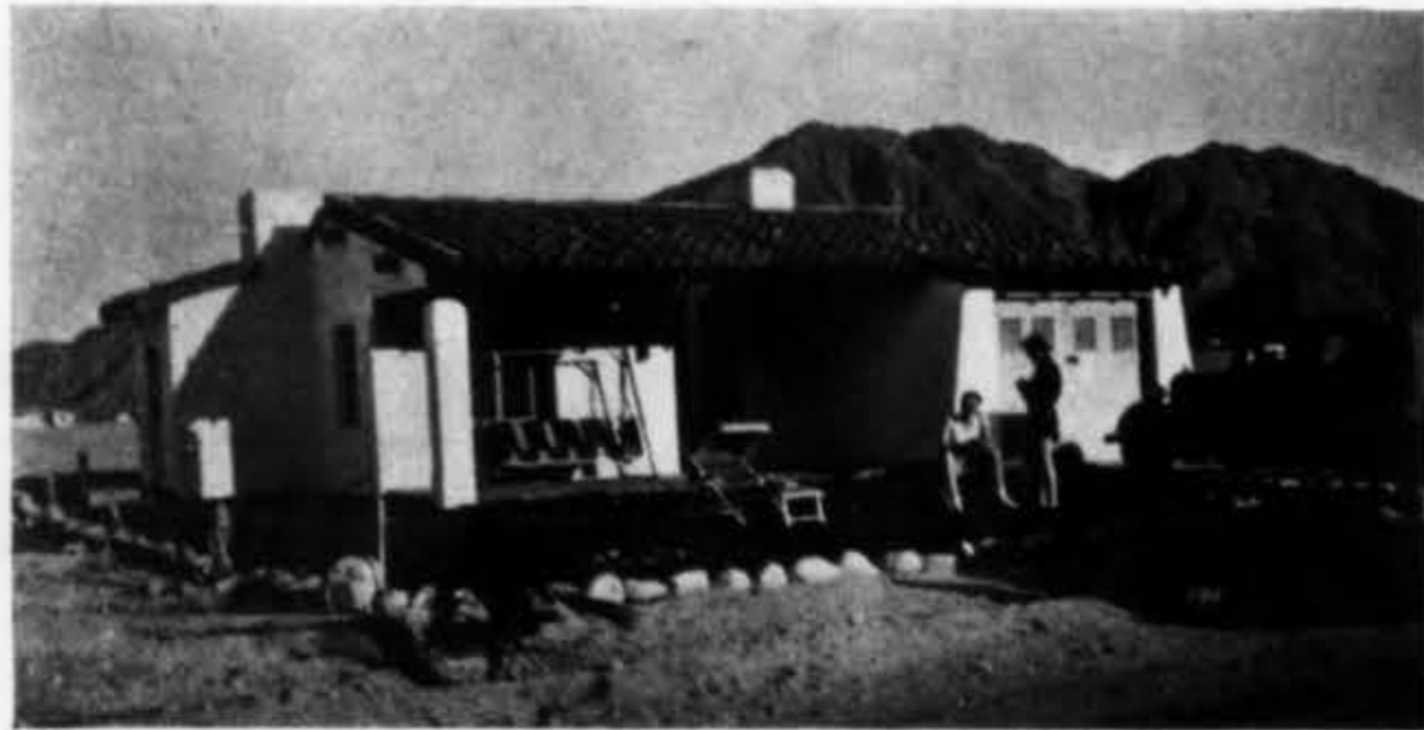
California concrete home constructed with our mortarless interlocking hollow blocks
