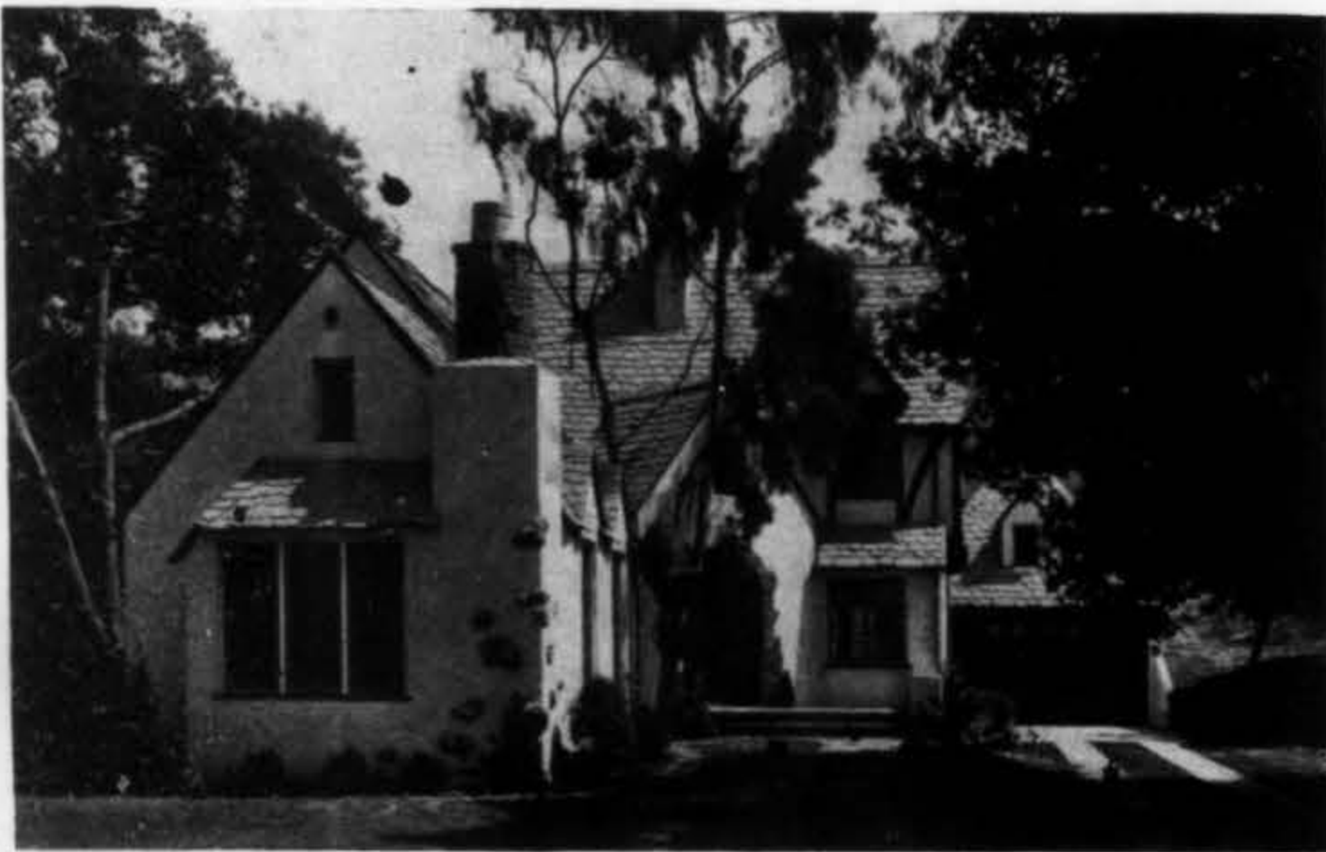
Here is a two-story English type house with steep roof. Built of wood frame and finished with cement stucco, the roof is covered with asbestos cement shingles.
