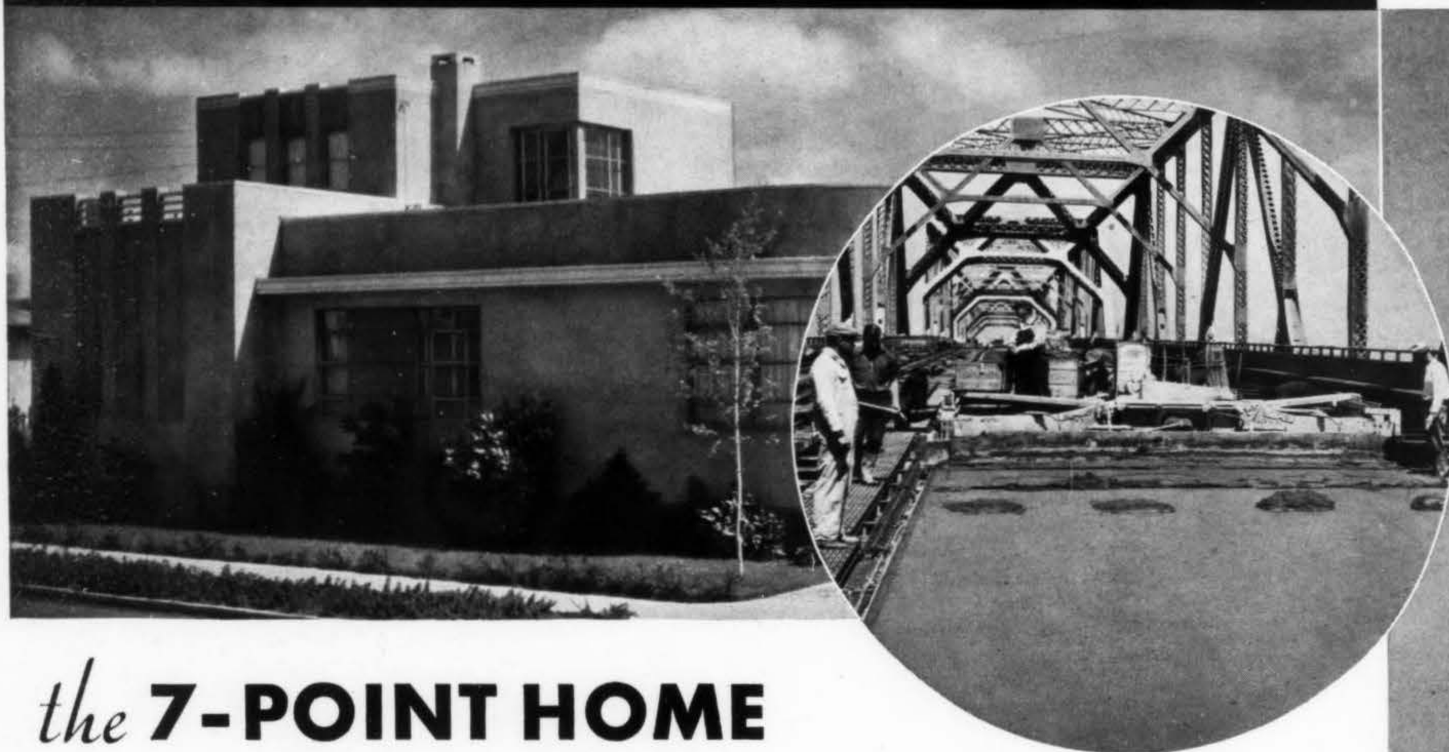
Gravelite concrete being poured in upper deck of San Francisco- Oakland Bay Bridge
