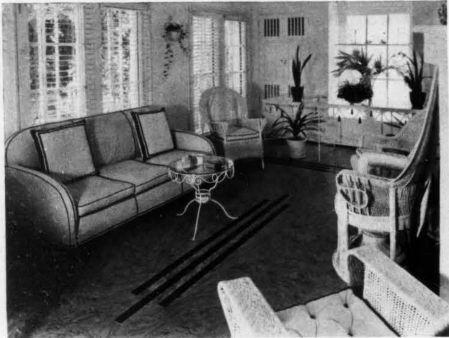
Plain or mottled colors of linoleum with strips or borders make it possible to secure original patterns and designs that are appropriate for most rooms of the house. This pattern in the sun room of a Hollywood residence is quite effective. Photograph courtesy of Armstrong Cork Products Company.
