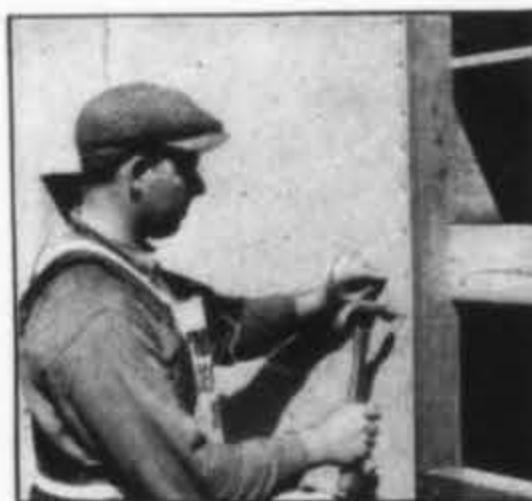
(Above) Millions of sealed air cells within the fibres of Celotex are a natural bar to heat transmission. Open network of strong Celotex fibres means increased air space—increased insulating efficiency.
