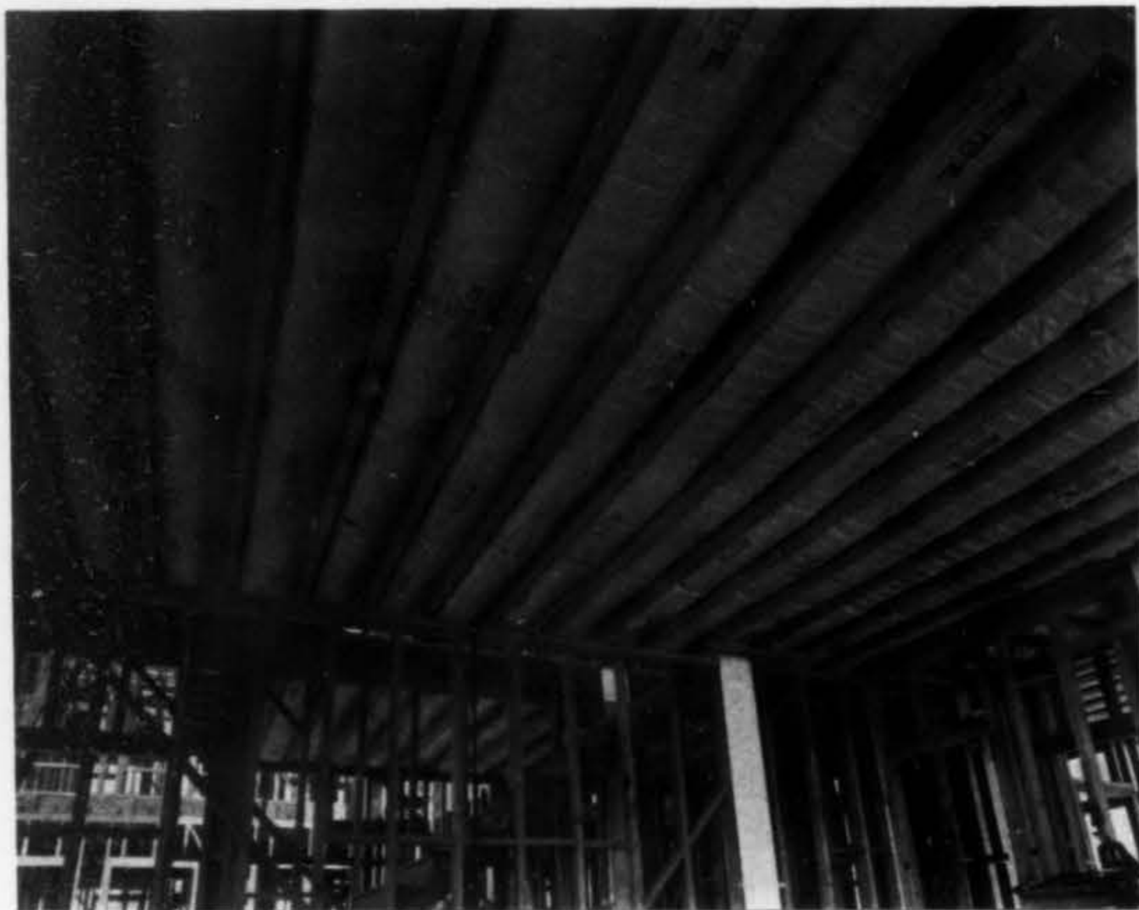
Photograph showing AllTite Insulating Quilt placed between second floor joists and suspended ceiling. See detail at right.
