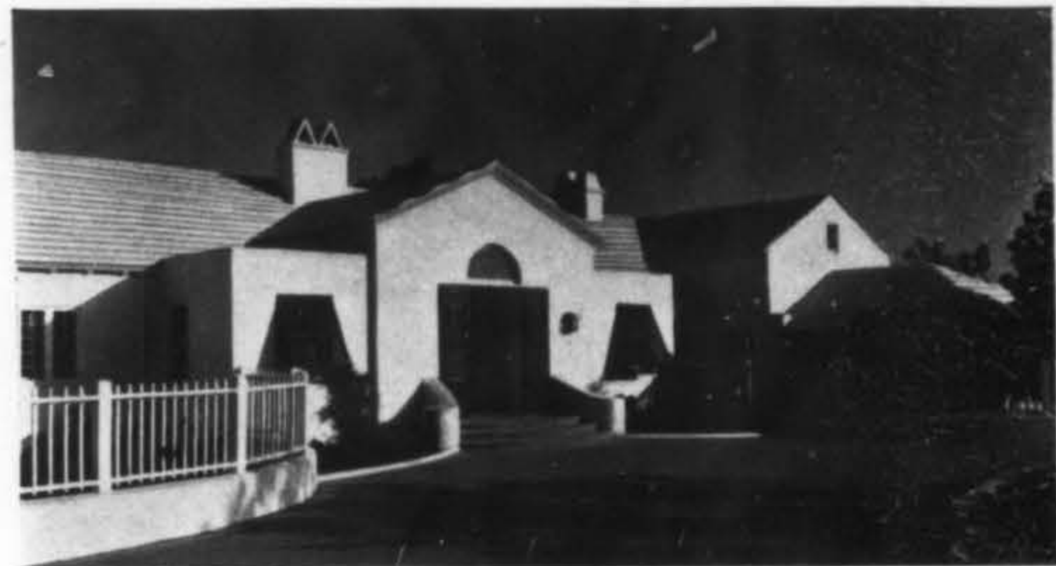
MR. AND MRS. GARY COOPER RESIDENCE ROLAND E. COATE, A. I. A. Associate Architect
