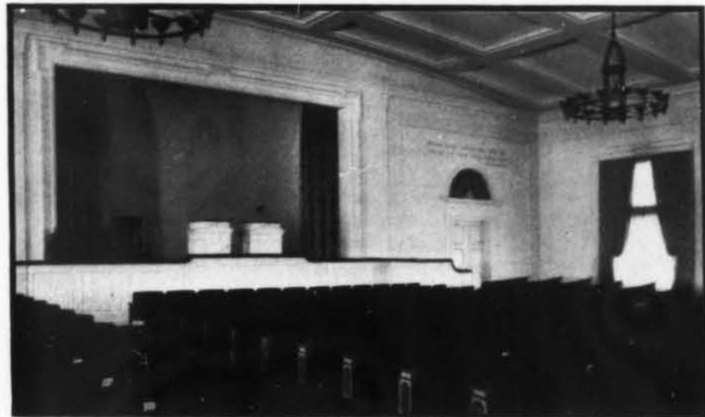
Twenty-fifth Church of Christ, Scientist, Los Angeles, H. Roy Kelley, Architect, is heated with three Payne "CB" Furnaces.
