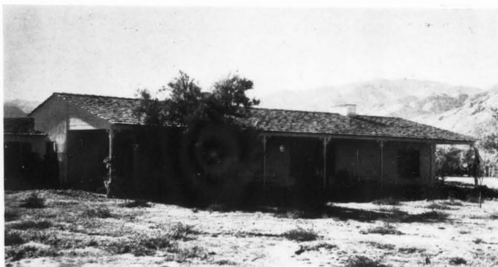
The ranch house of Mrs. M. J. Harrison at Palm Springs has two diagonal wings which form a large patio with a separate house for the complete comfort of guests. The living room opens into the patio through a large sliding glass door. Mrs. Harrison has furnished the house with furniture collected in the Philippines. Van Pelt and Lind, architects.
