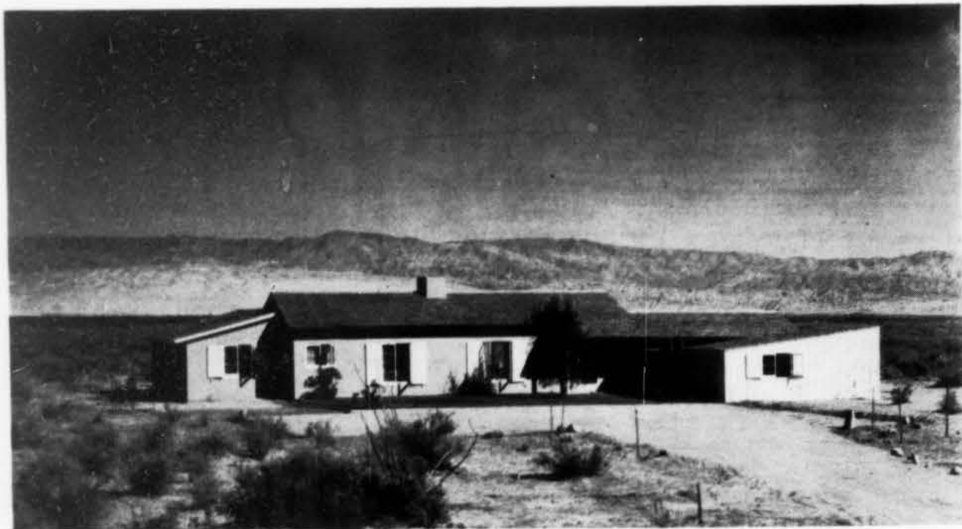
The Palm Springs home of Mr. and Mrs. Alger Shelden is built of cement block walls painted an Indian red, with white wood sash, and a wood shingle roof left natural. The living room and patio are on the opposite side to the approach, thereby assuring privacy from the road and lookout over the desert. Van Pelt and Lind, architects.
