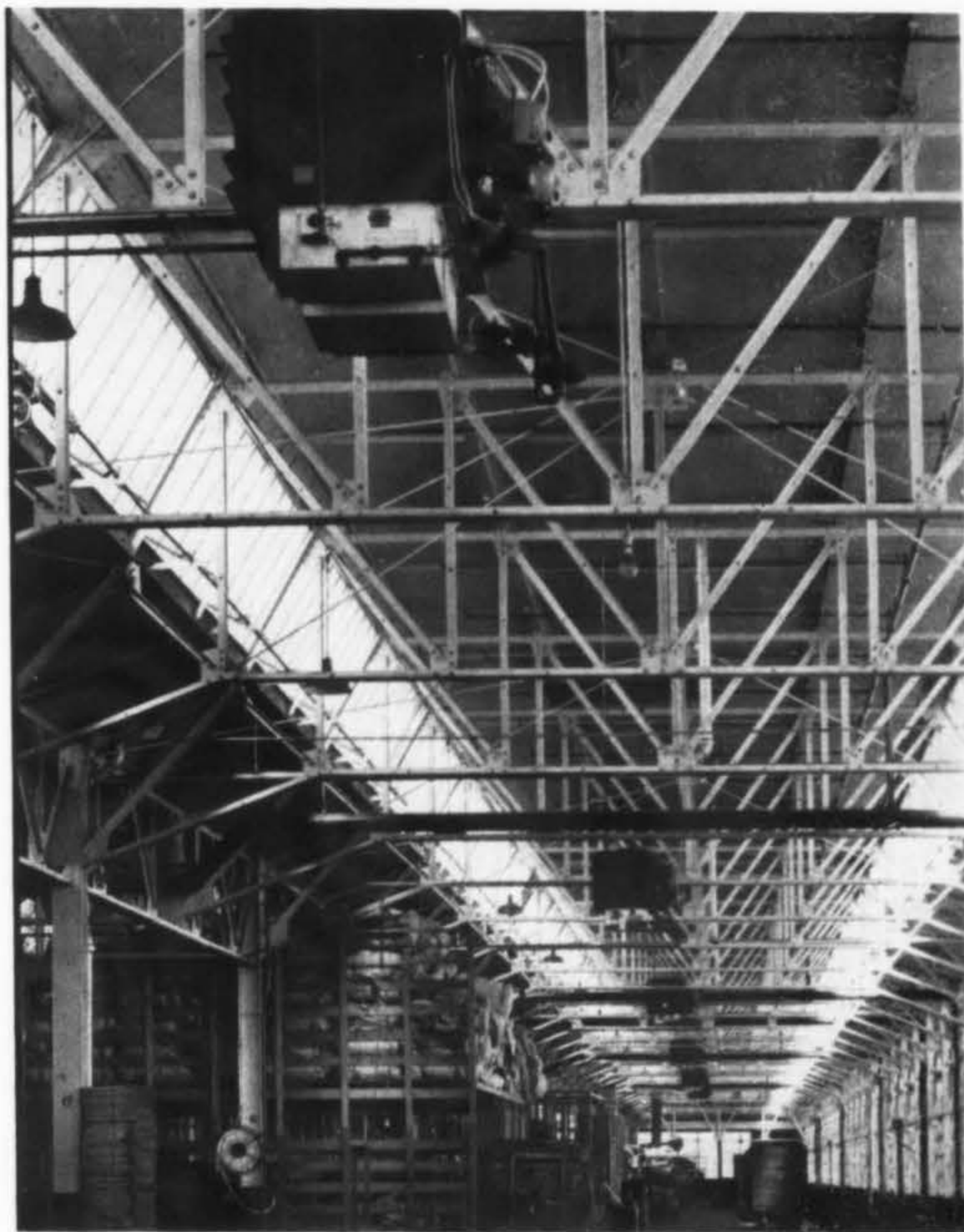
East bay of the General Motors Assembly Building showing Pacific Overhead Heating Units.
