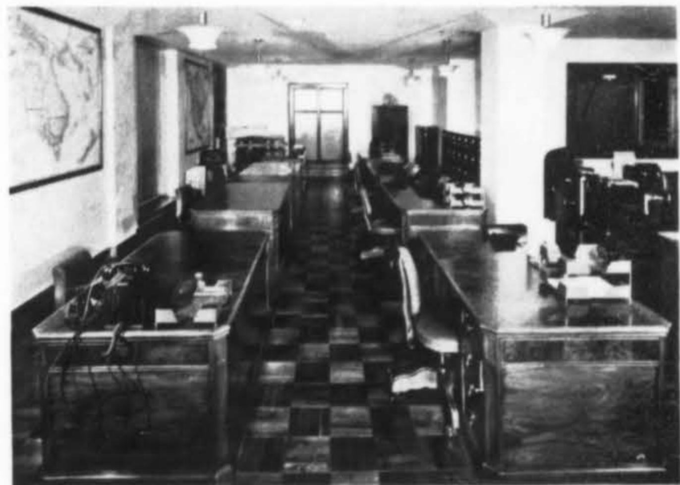
Walnut block floor laid in mastic on concrete in offices of Max Factor & Co. in Hollywood. Executed by L. D. Reeder Co.
