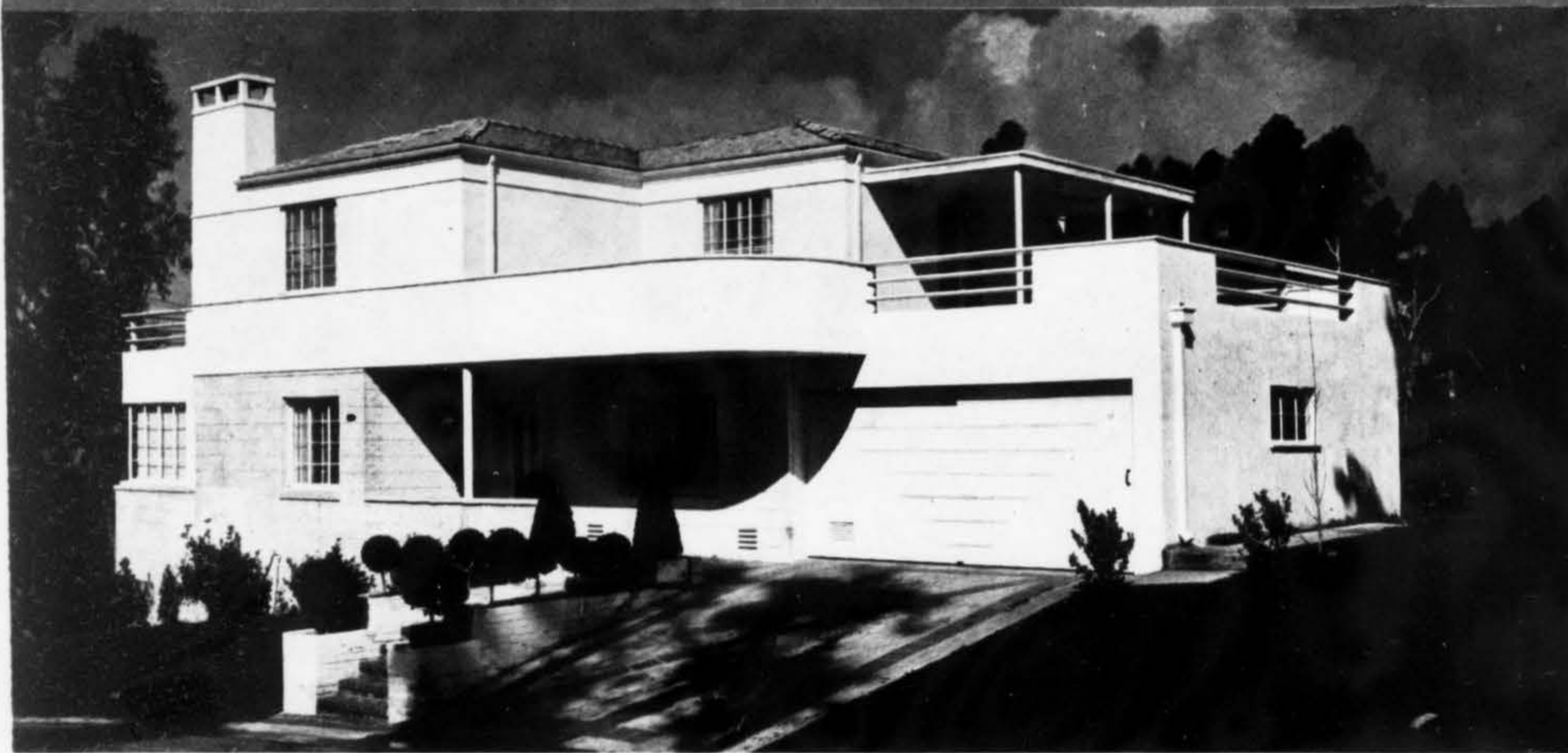
General Electric Model Home, Berkeley, California. John Ekin Dinwiddie, Architect J. M. Walker, Builder
