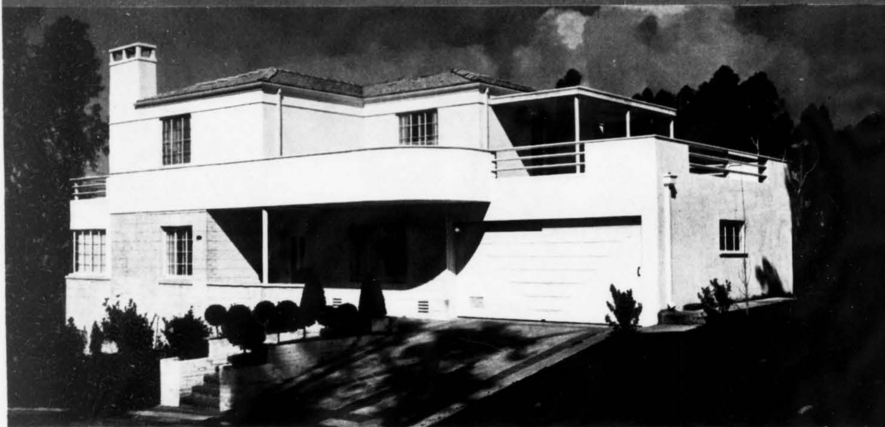
General Electric Model Home, Berkeley, California. John Ekin Dinwiddie, Architect J. M. Walker, Builder
