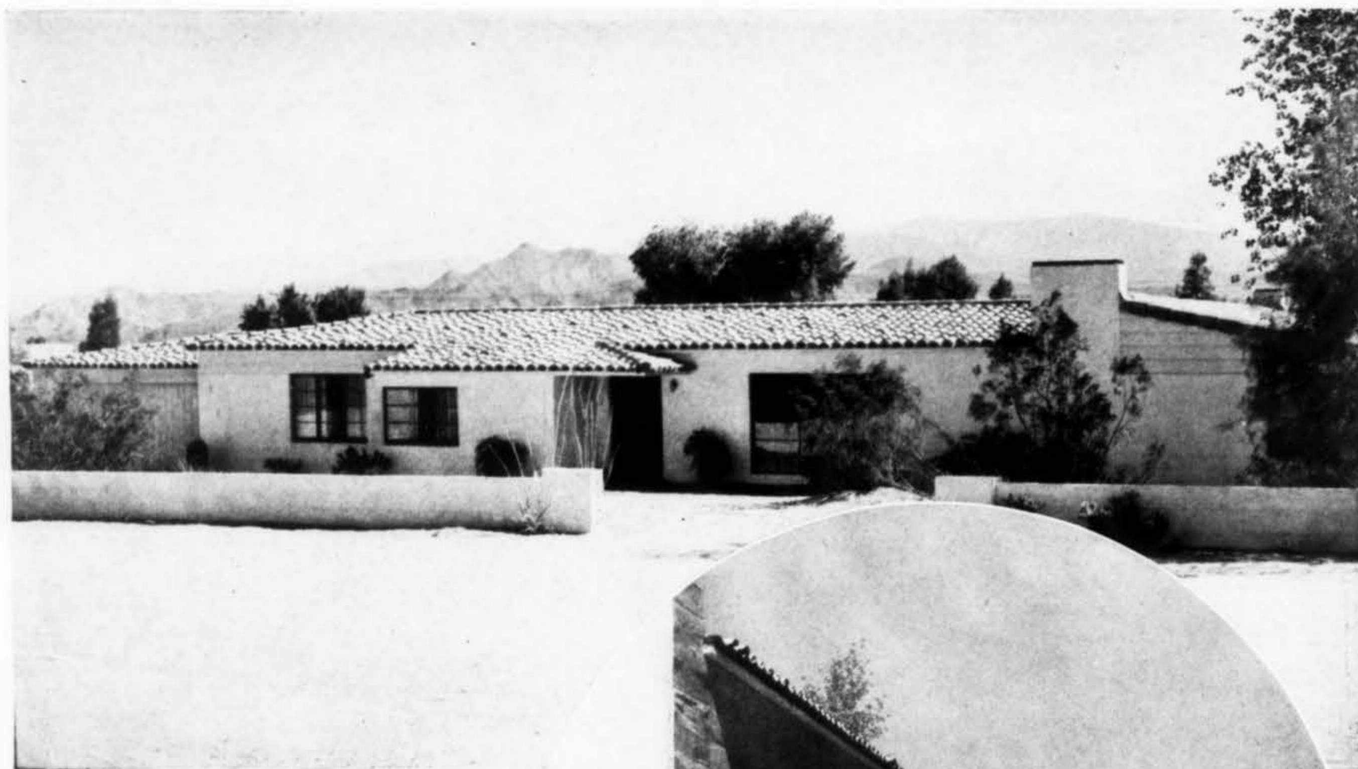
Residence of Thomas Slaven at Palm Springs, California. Designed and built by Van Evera Bailey. Monolithic concrete construction with hollow concrete walls. Typical of the homes which helped establish an all-time high for concrete in 1936 through America, both in number of homes built and in percentage of the residence market.
