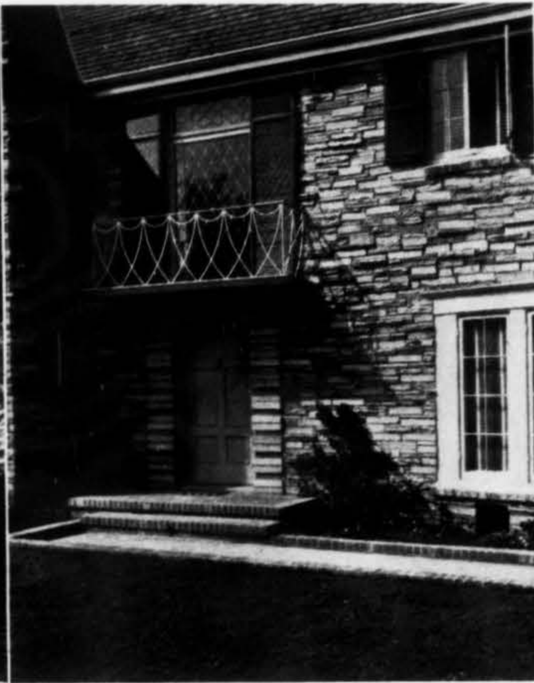
In the center the home of Dr. and Mrs. Barney Kully designed by Architect Heth Wharton has a concrete masonry veneer closely resembling field stone and lending an air of solid and substantial dignity.
