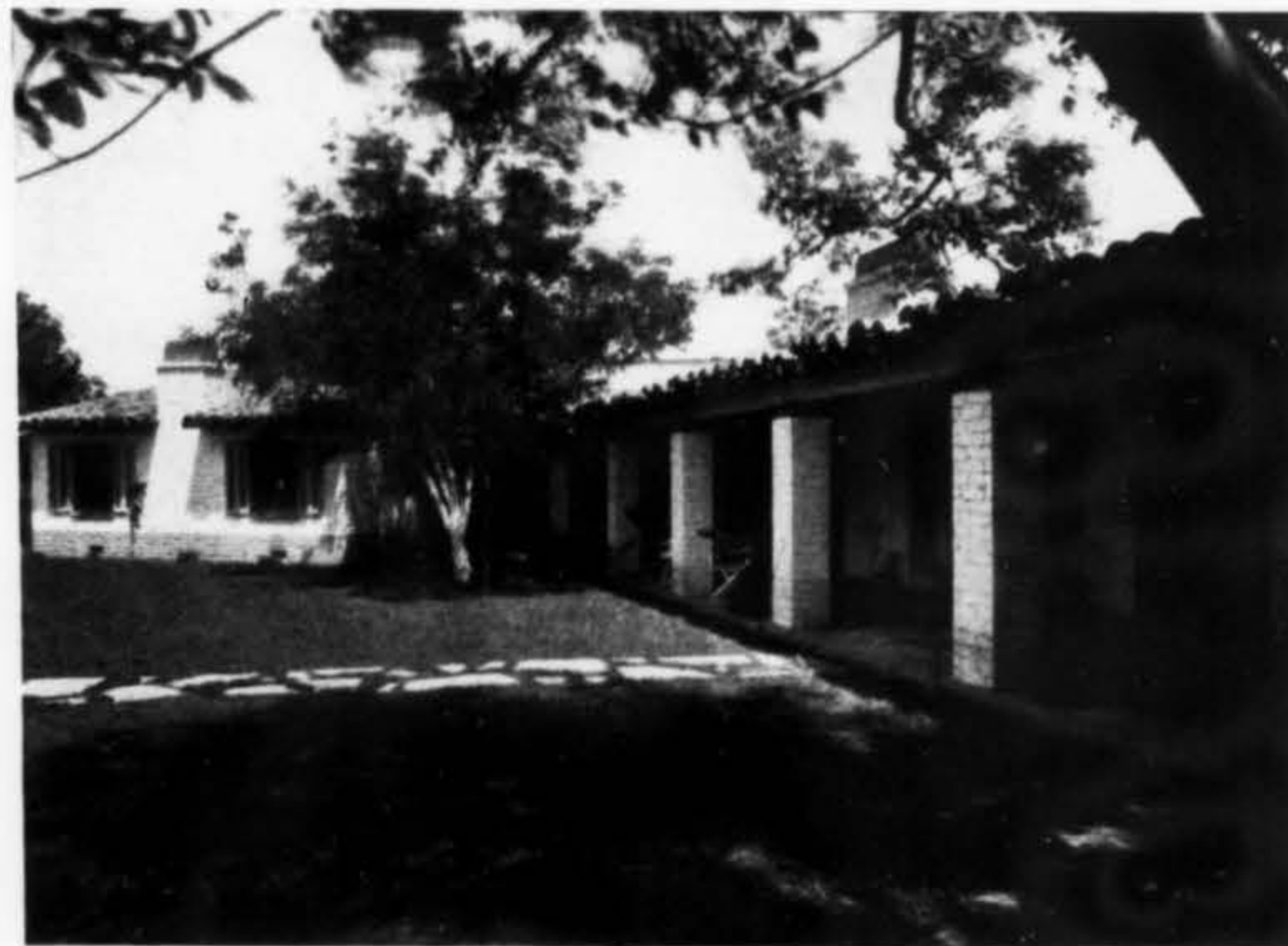
Residence of Mr. and Mrs. Seton I. Miller Van Nuys, California CHARLES O. MATCHAM, Architect
