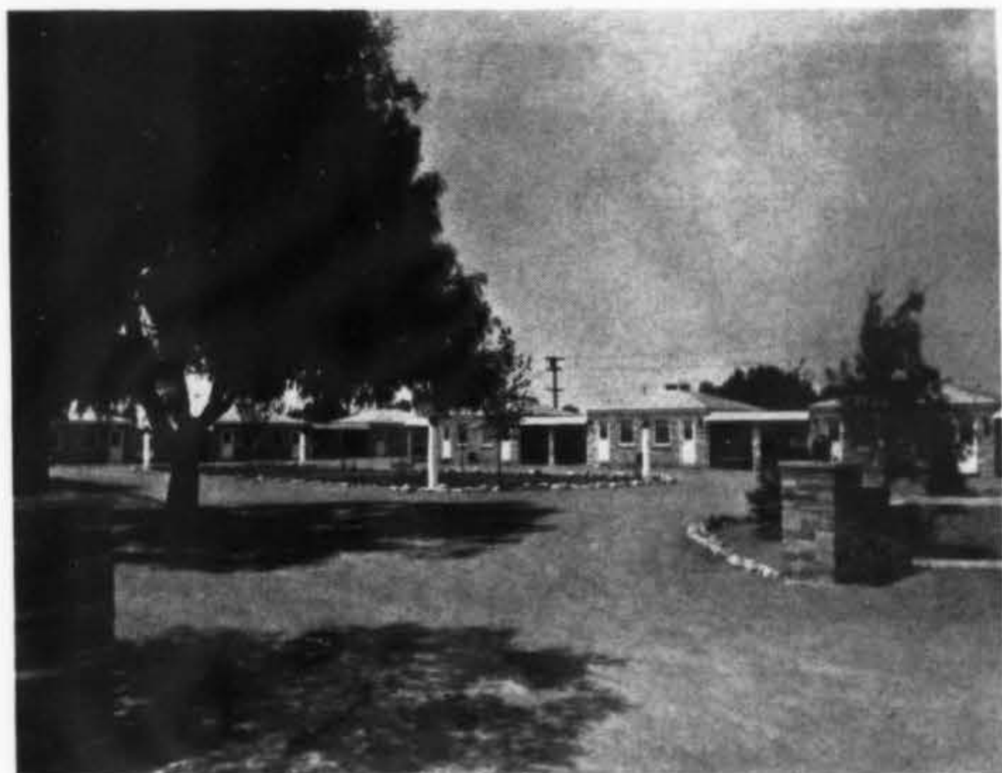
An auto court that answers a motorist's prayer. Clean, comfy and substantial—quite—with solid masonry walls eight inches thick reenforced by solid concrete studs. The interiors left unplastered have been painted in soft colors guaranteed to bring sweet dreams.
