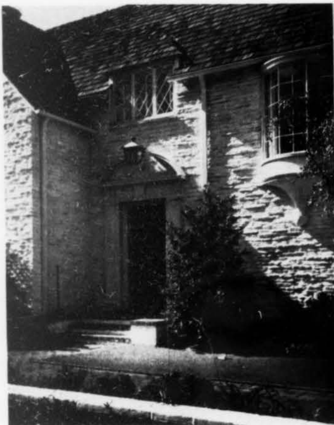
Three doorways in the concrete manner. On the left an entrance designed by Architect H. Roy Kelley. Masonry walls of random ashlar "slump" have been painted to give a surprising richness of texture.
