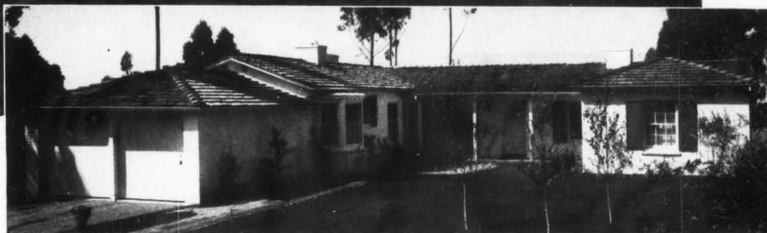
Residence of Mr. and Mrs. Vernon Ball, Creston Road, Berkeley. Edwin Lewis Snyder, Architect; J. M. Walker, Builder.
