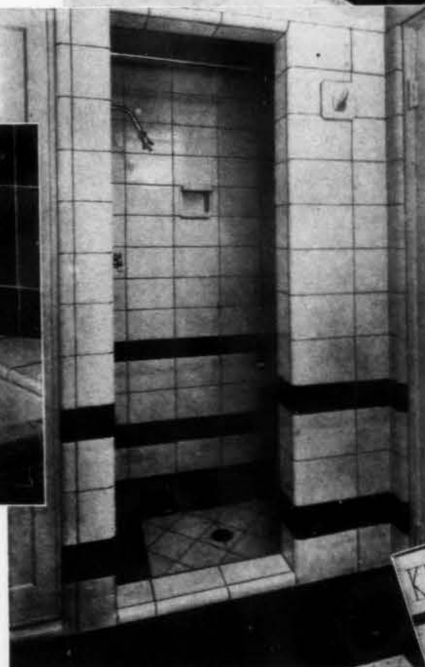
A particularly interesting Master Kraftile treatment for a modern all-tile shower. Here cream tiling with horizontal bands of black show off to splendid advantage how effectively 6 x 9 Master Kraftile makes the smallest room appear more spacious
