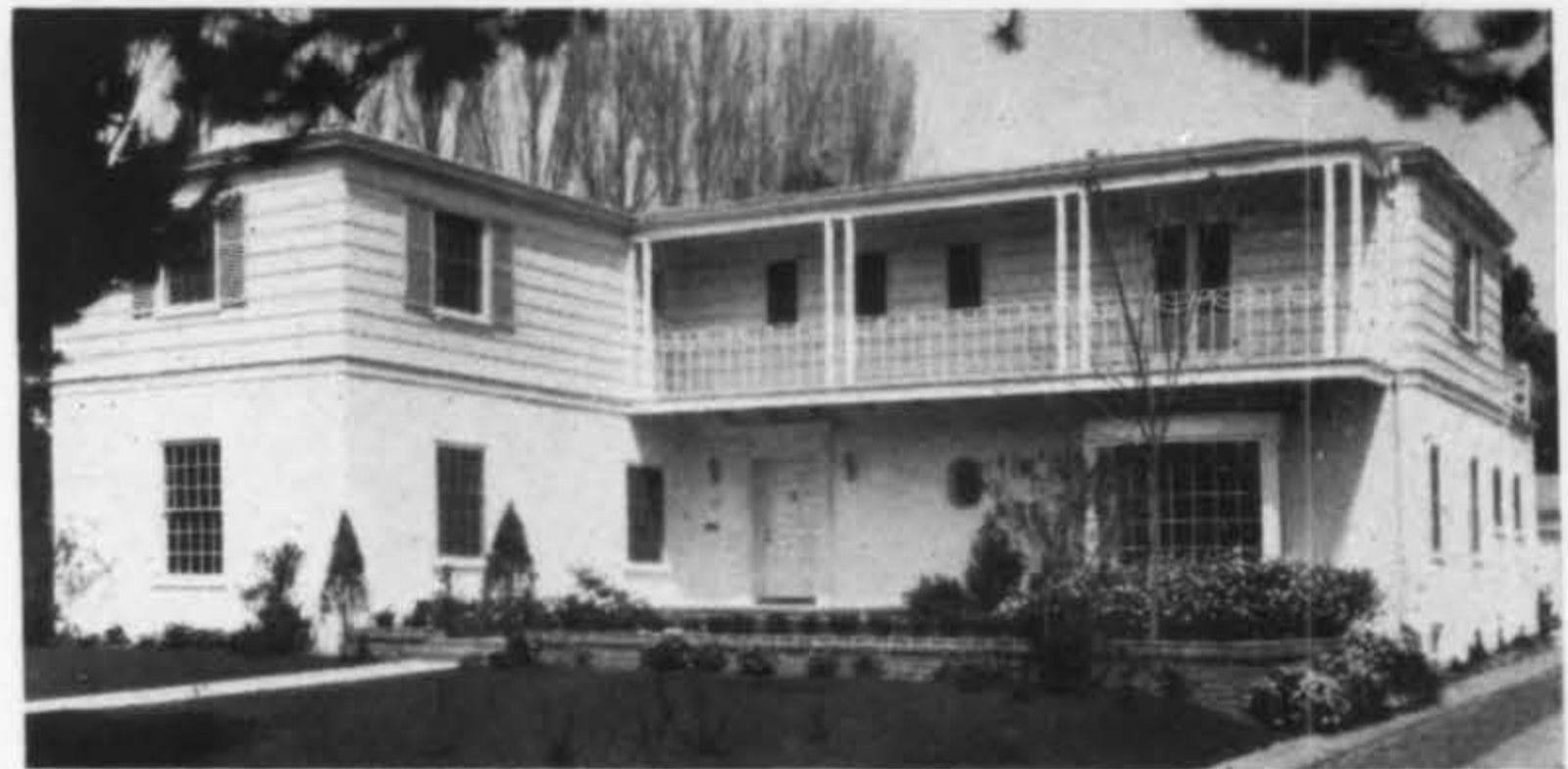
PAYNEHEATED RESIDENCE DESIGNED BY HOWARD G. ELWELL AND ARTHUR L. HERBERGER, ARCHITECTS
