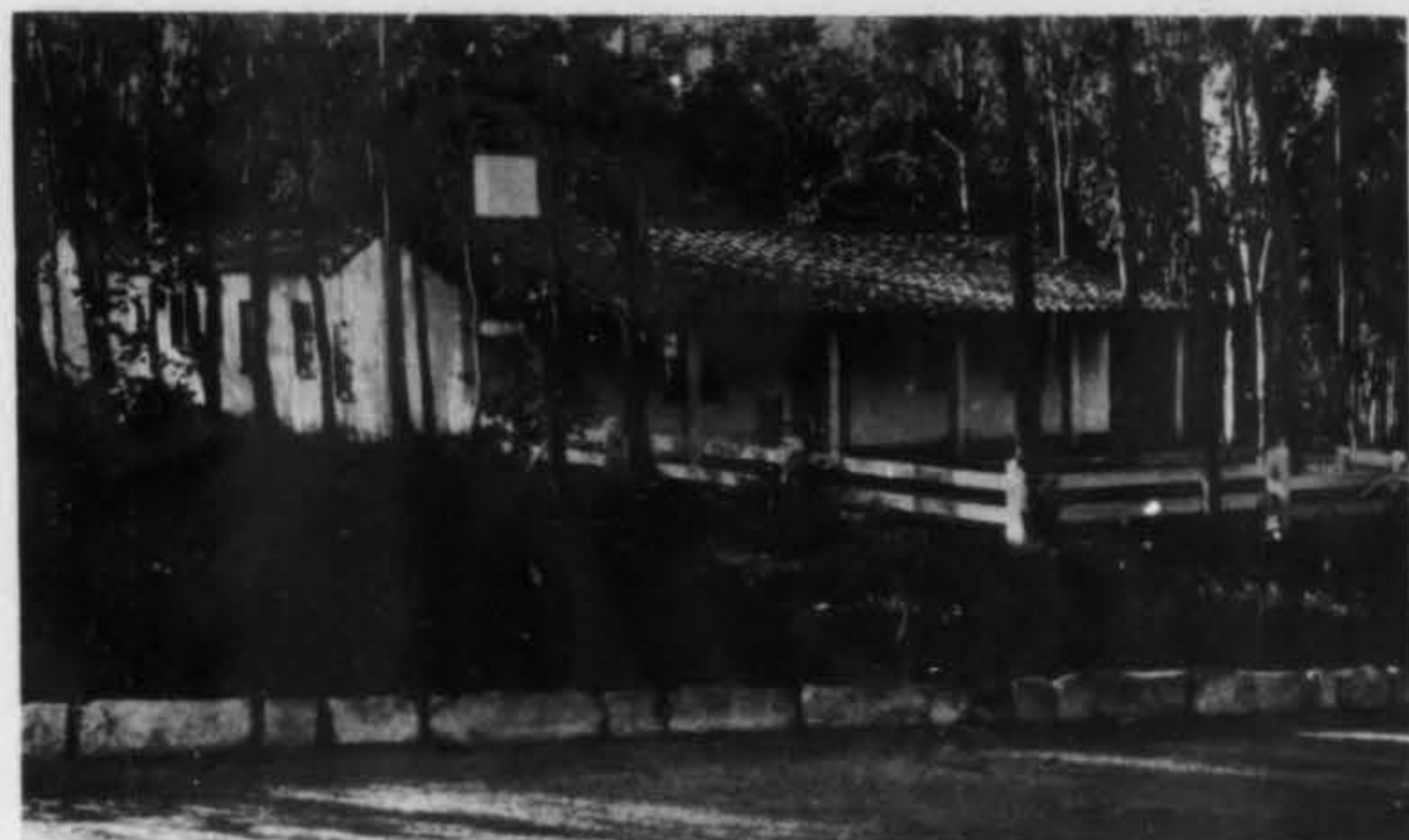
HERBERT C. HOWARD, ARCHITECT V. C. SMITH, BUILDER
