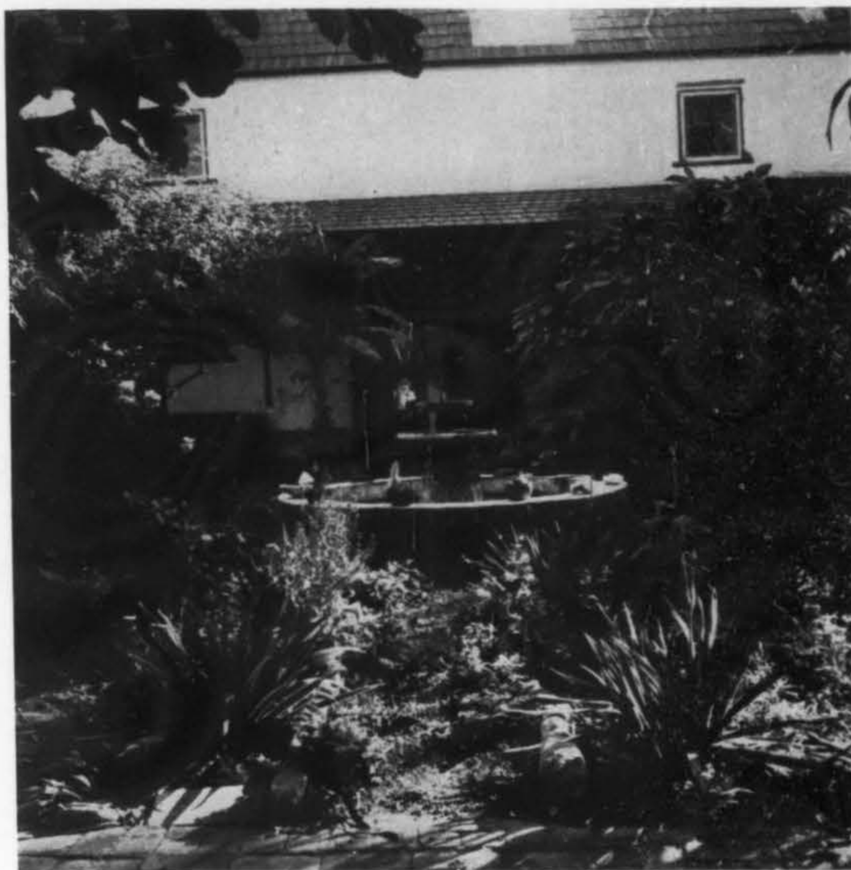
The patio with its fountain is a Spanish retreat of coolness, flowers and water, its overgrown informality giving it added charm and picturesqueness. Below, the restoration in progress. Note the patches of original plaster and the wooden binding plate which runs along the outside wall.
