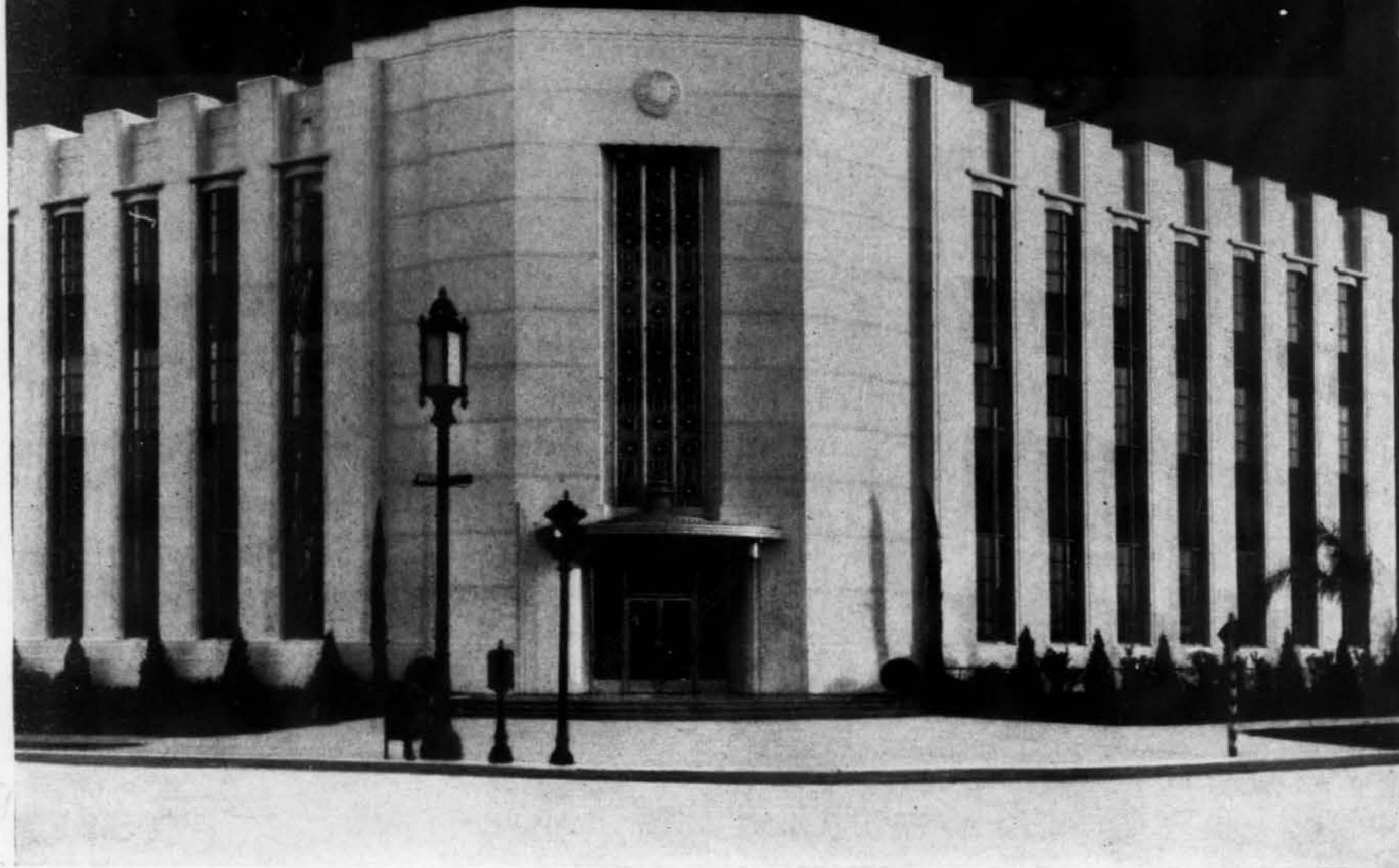
Farmers Insurance Company building at 4680 Wilshire Boulevard, Los Angeles. An outstanding structure on a street of fine buildings. Walker and Eisen of Los Angeles, architects; William Simpson Construction Co., contractor.
