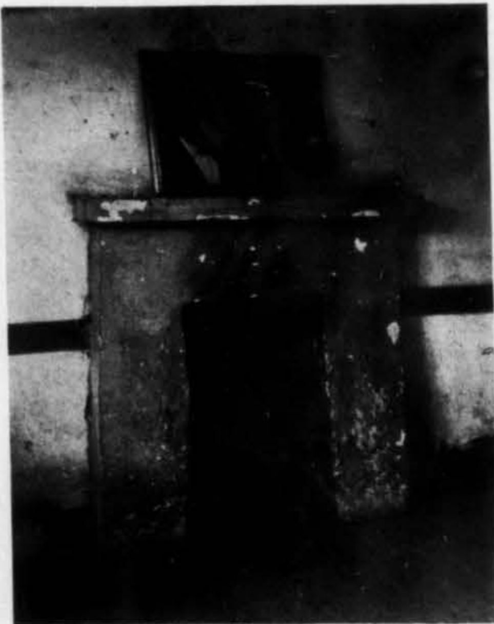
A fireplace in the mansion of Don Pio Pico built for logs to be placed upright.
