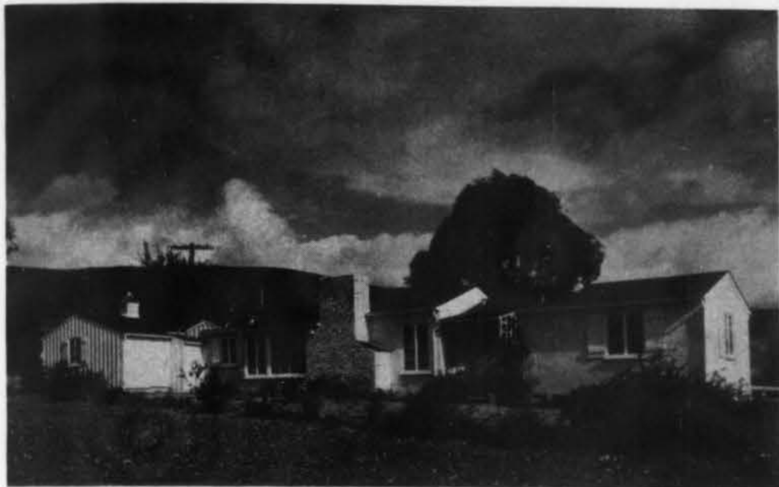
THE RESIDENCE OF MR. AND MRS. W. GLENN WELLS at Three-Arch Bay, California CHARLES A. HUNTER, A.I.A., Architect
