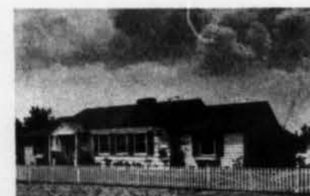
Front view, Redwood picket fence
