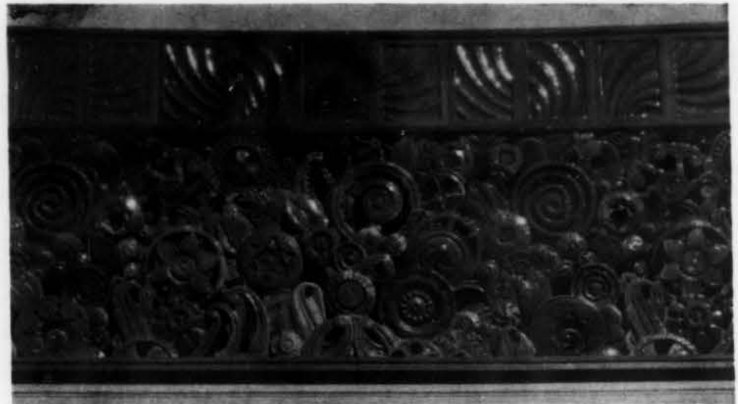
An open work panel six feet deep in jade green tile forming a frieze of delicate design across a building. Of hand-made terra cotta, much the same methods were used as were used hundreds of years ago. Courtesy of Gladding, McBean & Company.
