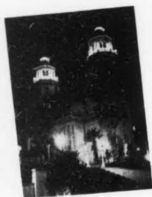
View of a small part of the famous William R. Hearst Castle at San Simeon where our sub-irrigation root system has saved many old oaks.
