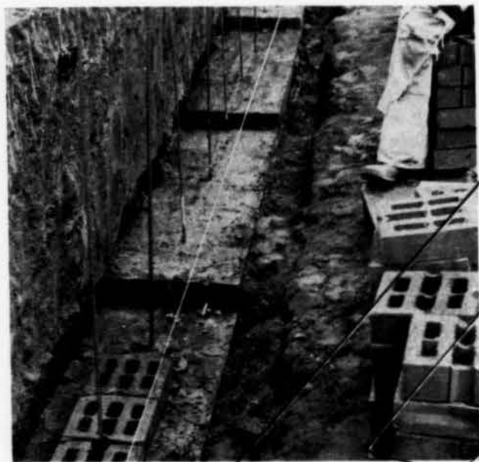
DOUBLE BRICK makes a simple, easy job of stepped or irregular foundations.
