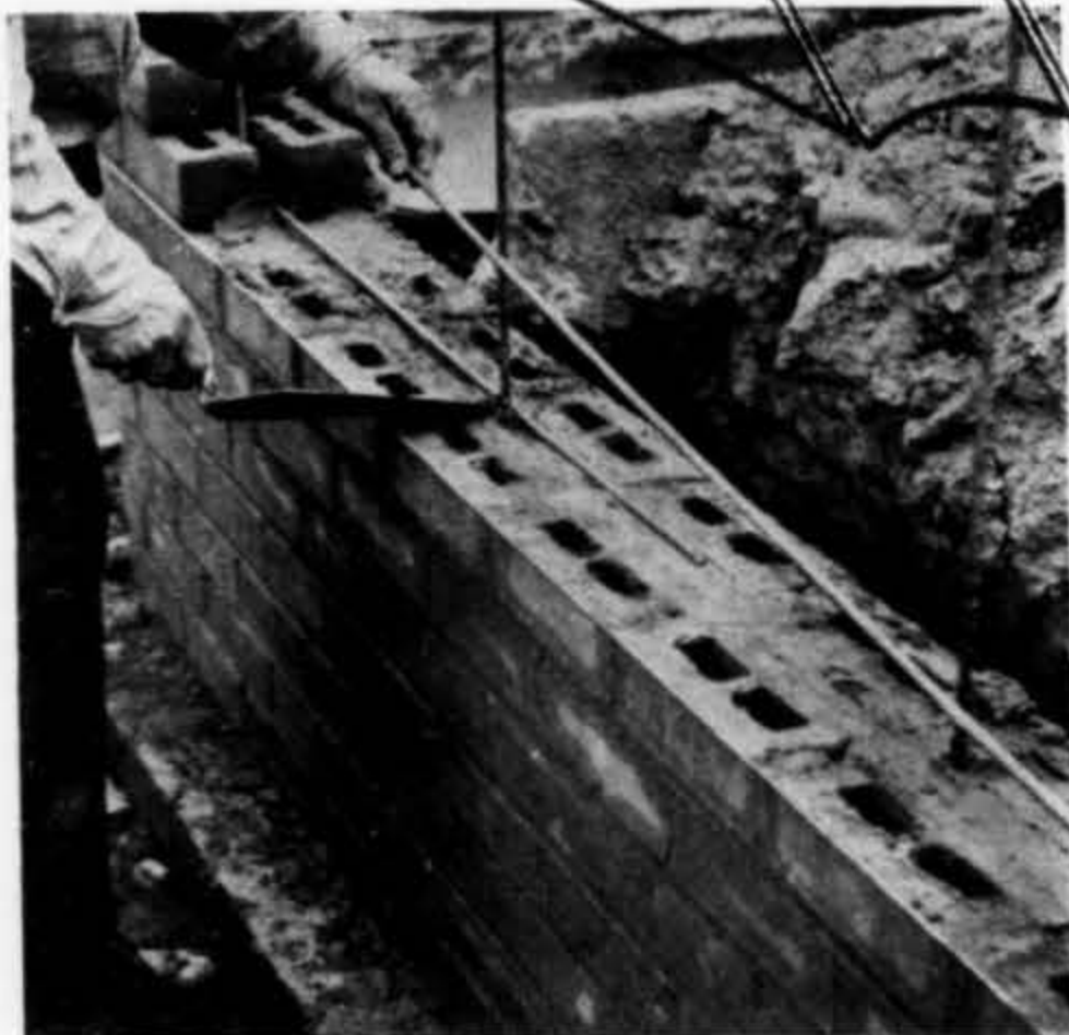
DOUBLE BRICK is easily reinforced. Steel rods "fit," both ways. No ties or anchors needed.
