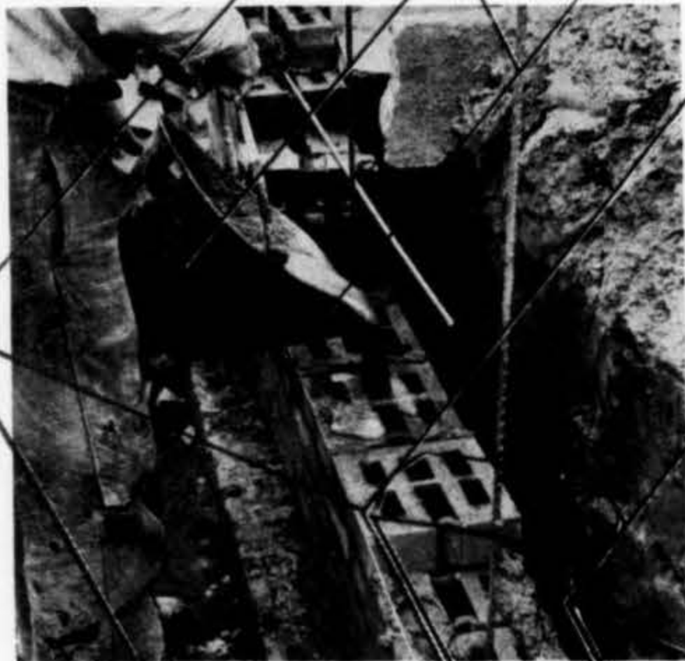
DOUBLE BRICK eliminates bracing, formwork. Prevents "spreading" when center voids are filled.
