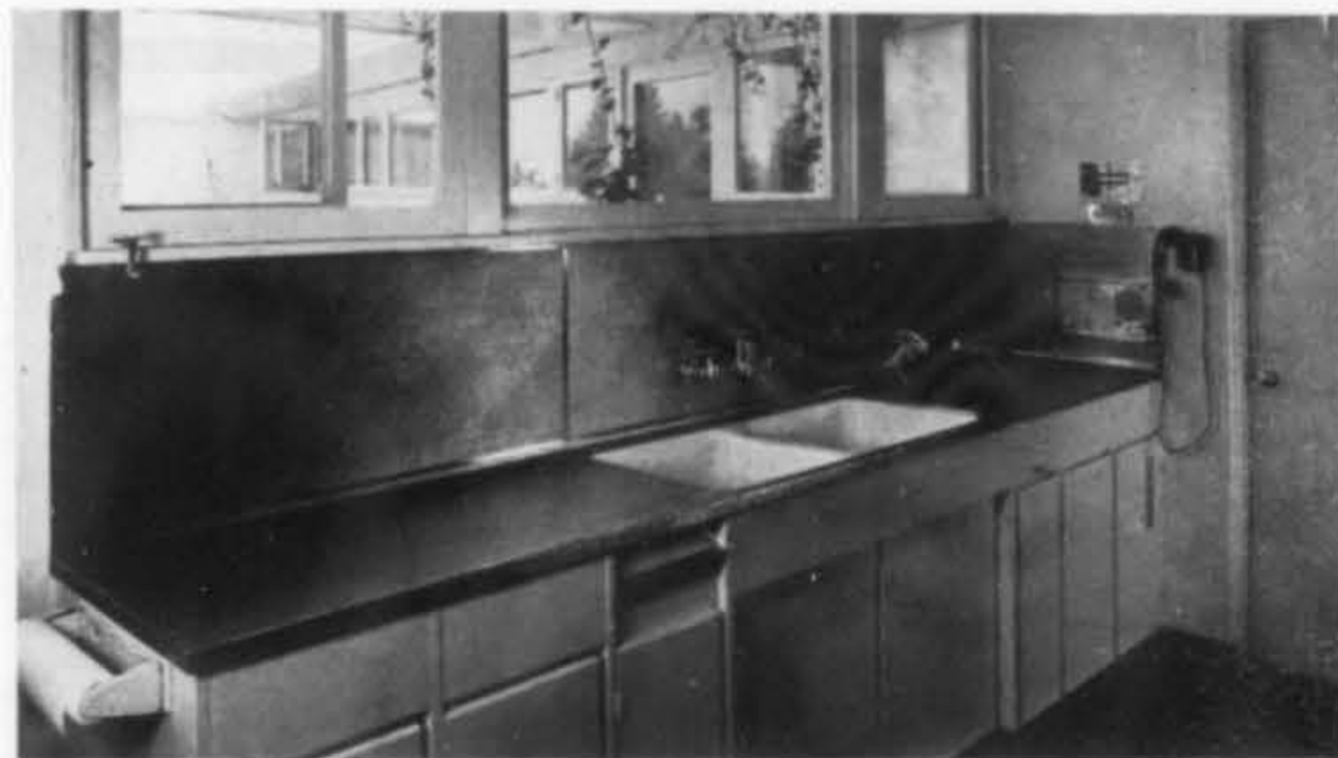
The drainboard and backsplash of LUDLITE Stainless Steel in the Berkson Houses . . . designed by J. R. DAVIDSON.
