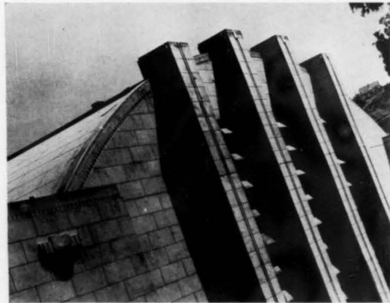
Giant pillars in martial rank of fours serve as impressive support for sides of the great drill hall
