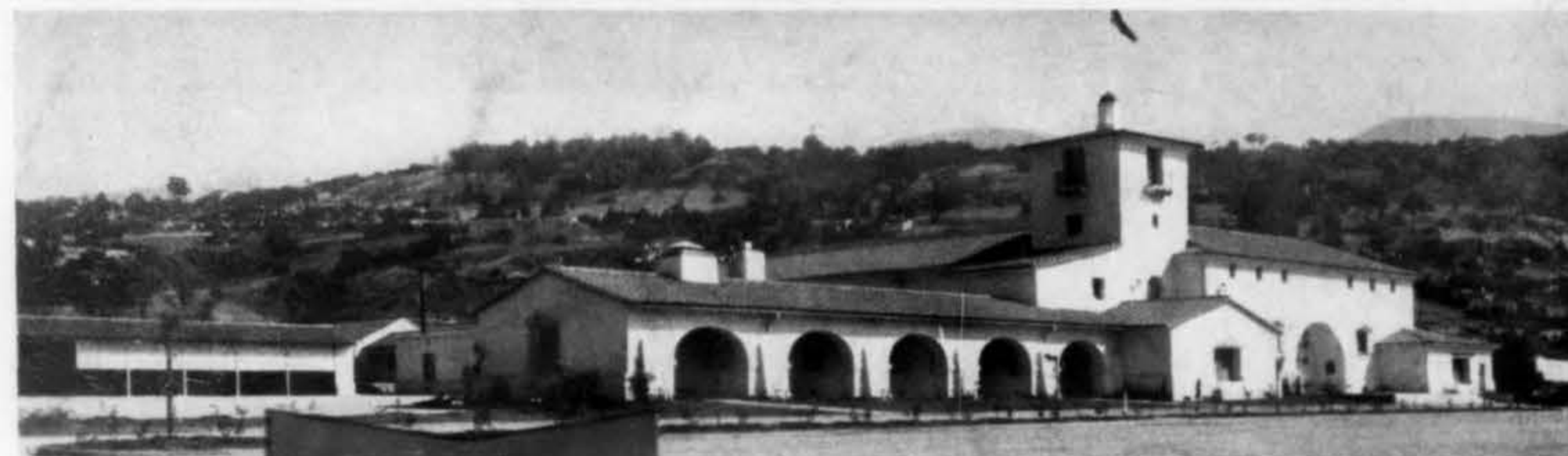
State armory for United States Treasury Dept., Santa Barbara, California. Drill hall covered by a Lamella roof, 93 foot span. Edwards & Plunkett, Architects. W. B. Coffey, Structural Eng.
