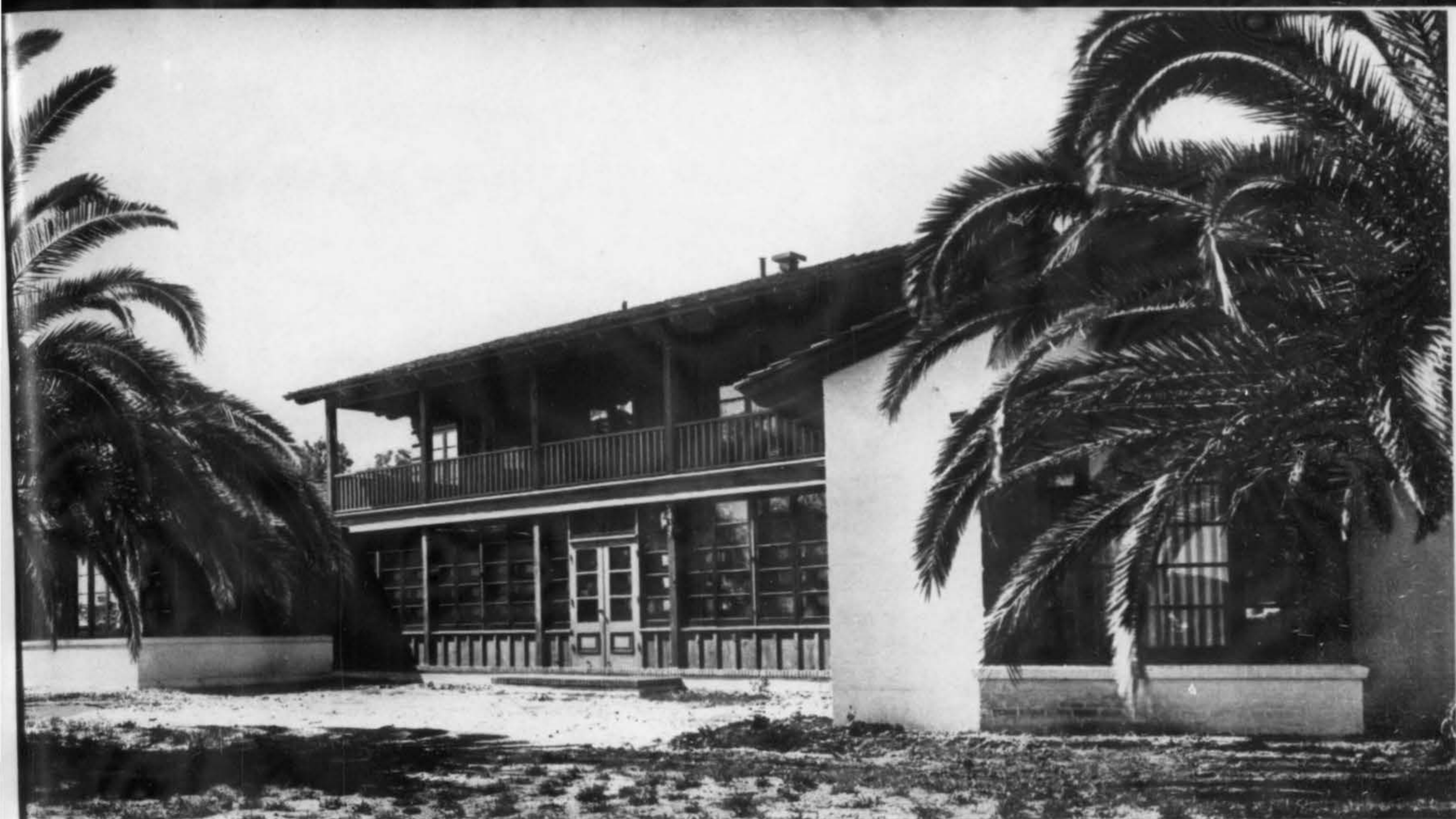
REAR OF THE HOUSE SHOWING THE ENTRANCE TO THE GLASS-ENCLOSED PORCH
