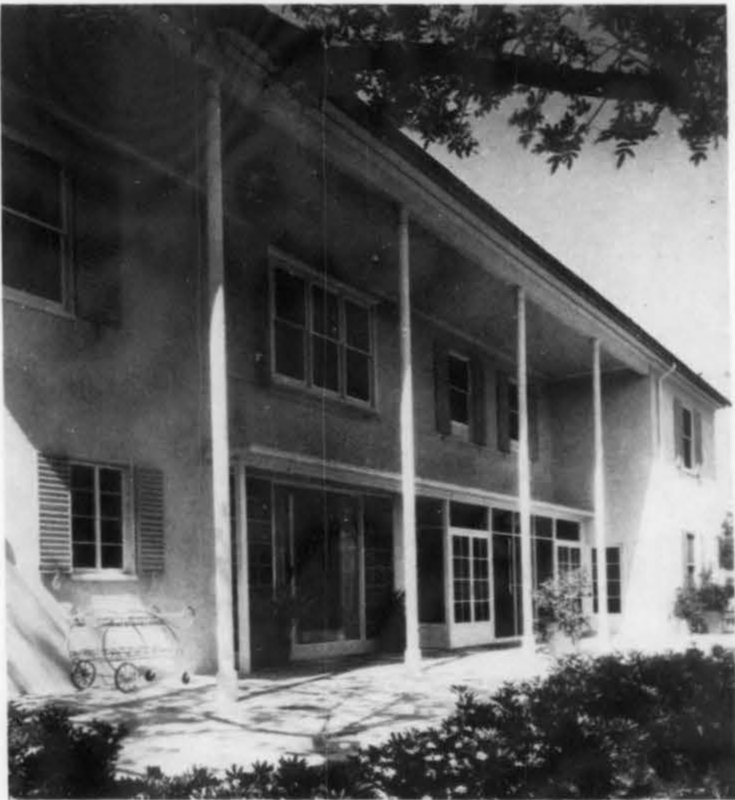
THE BROAD NORTH TERRACE AFFORDS AN ENTRANCE TO THE DINING ROOM
