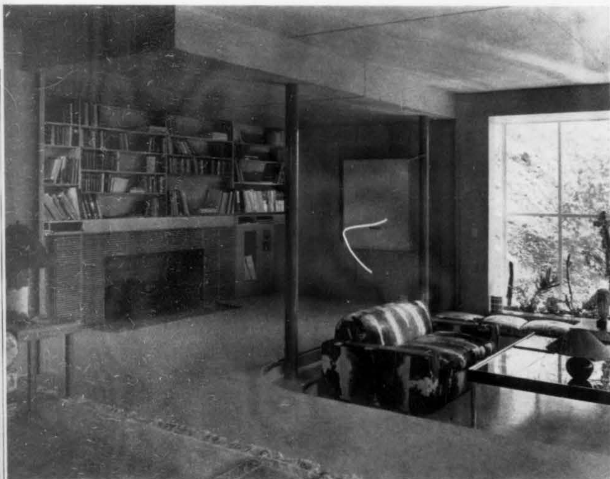
Living room detail showing red lacquered steel columns and steps
