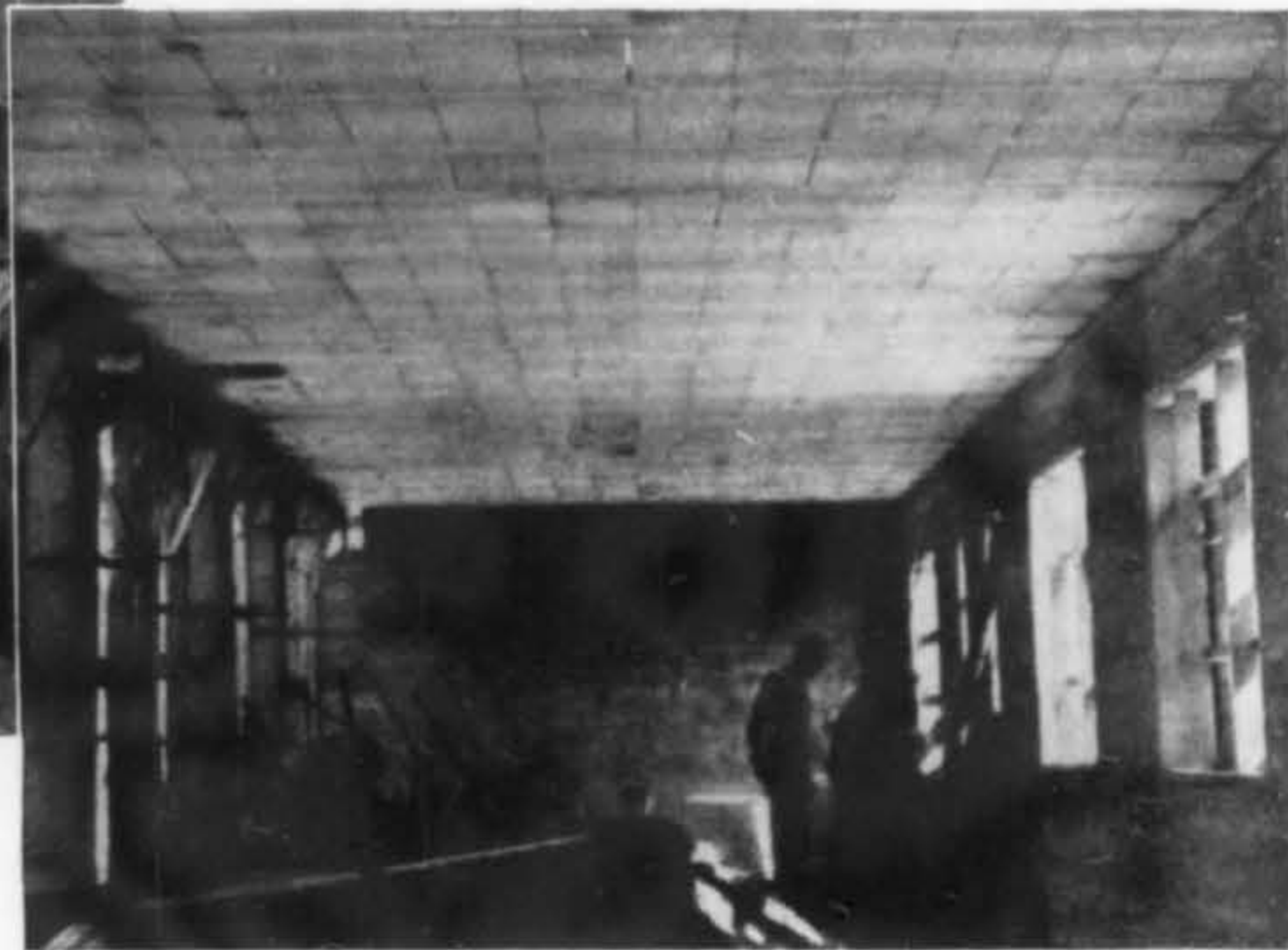
Above, light weight STANDARD Structural Gypsum poured over one section of girders. Right, ceiling of SIERRA Gypsum Tile and Structural Gypsum after plank forms removed.
