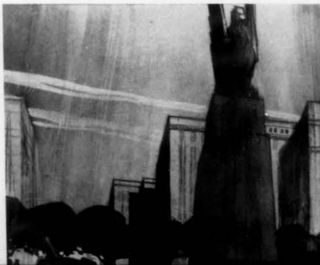
PYLON AT THE TUNNEL ENTRANCE OF BROADWAY
