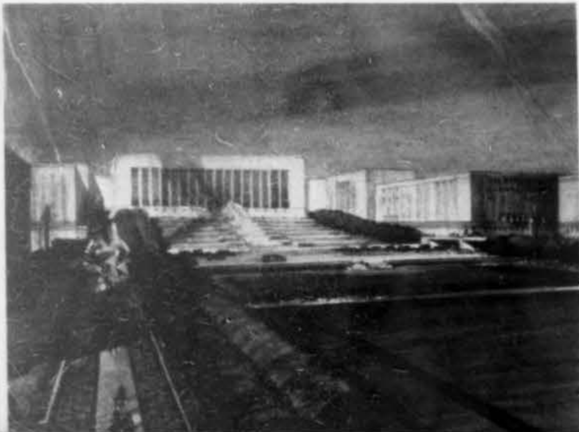
WESTERLY VIEW OF THE WATER AND POWER BUILDING
