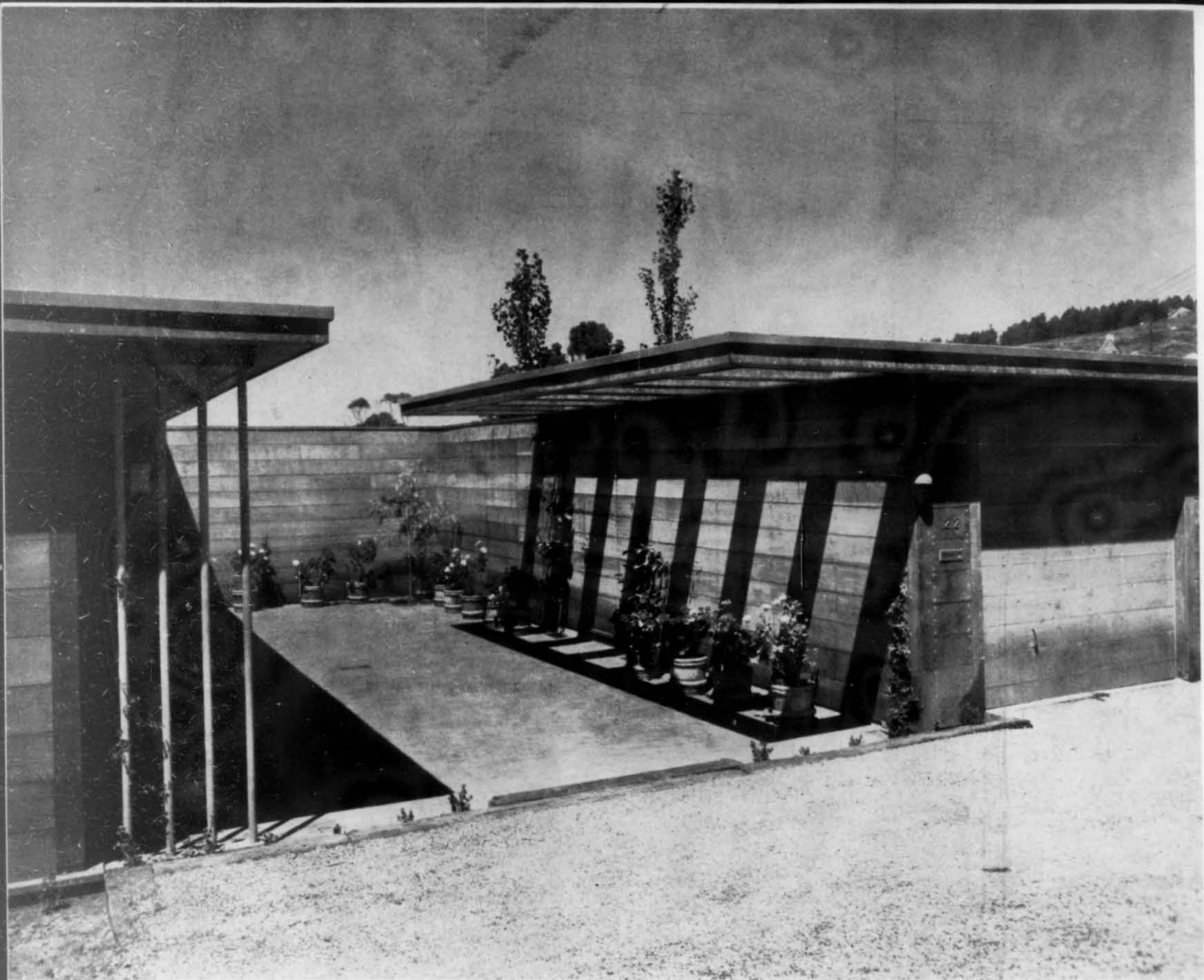
THE GARAGE IS PLACED IN THE CORNER OF THE ODDLY-SHAPED LOT AND IS CONNECTED TO THE HOUSE WITH A WALL WHICH FORMS THE ENTRY COURT
