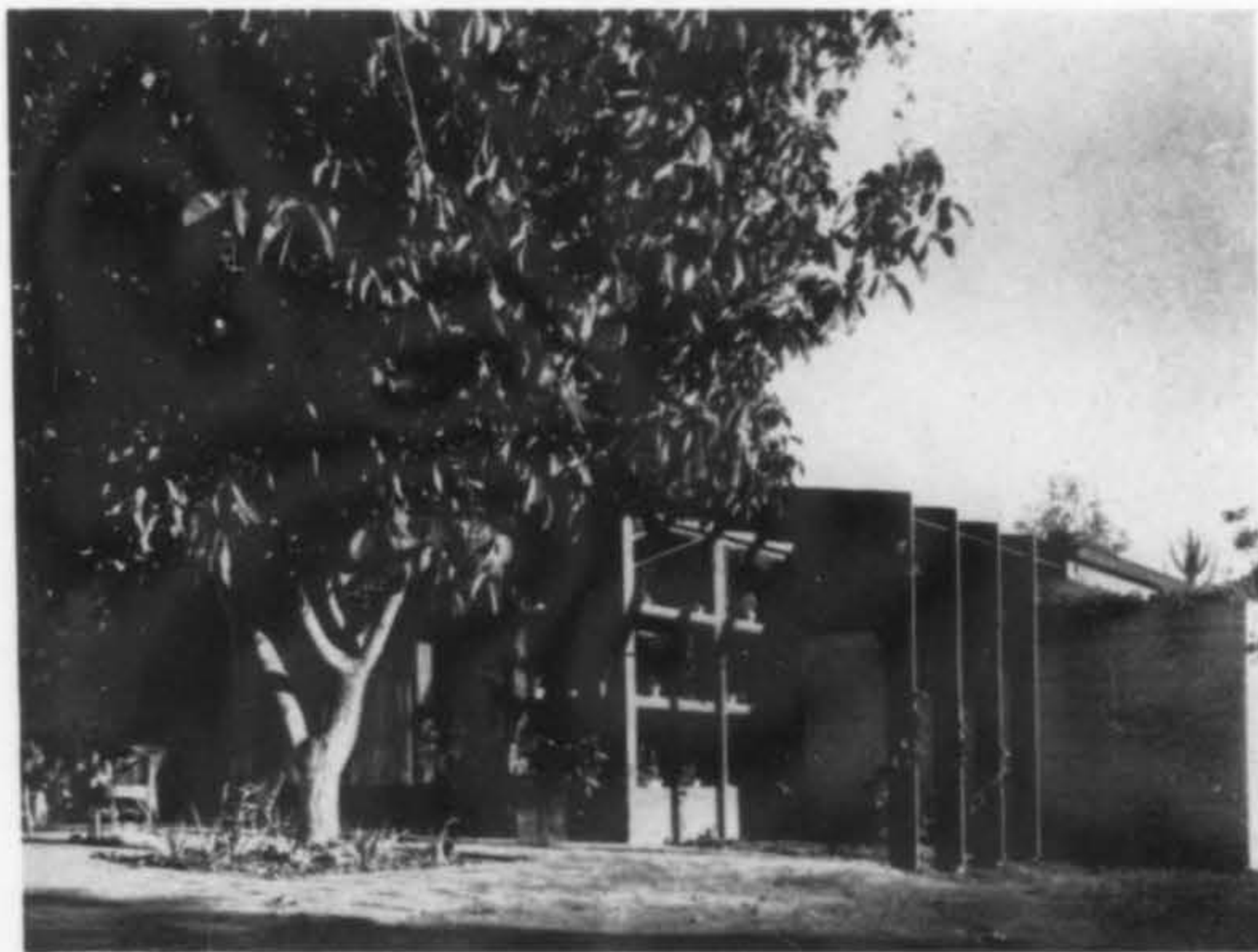
A VERTICAL TRELLIS, SCREENS THE WINDOWS ON THE WEST SIDE OF THE HOUSE
