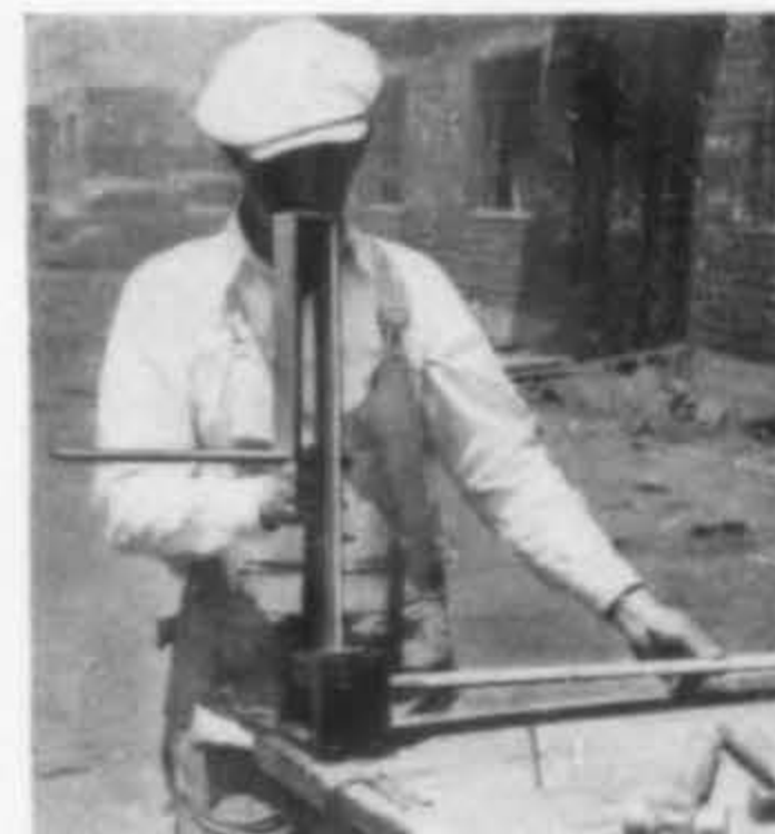
DEVELOPED BY GOLD BOND—No need for factory-cut units with Gold Bond metal base. Special cutting and bending equipment is supplied at low rental. Most complicated job conditions worked out on the spot. Contractor Fred W. Lorenz found this of great importance on the Carmelitos job.
