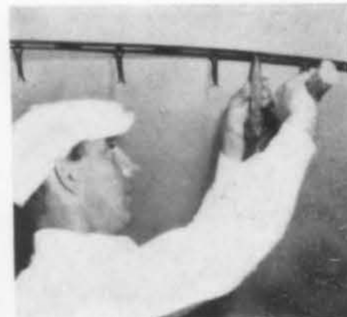
DEVELOPED BY GOLD BOND—Prong top runners go up quickly. Vertical prong rigid and long enough to allow for ceiling height variations. Prongs factory-spaced to meet any job requirement.
