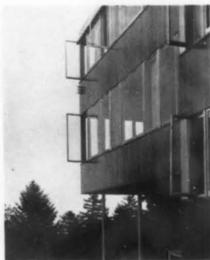
HARDWOOD SASH FOR DOUBLE GLAZING
