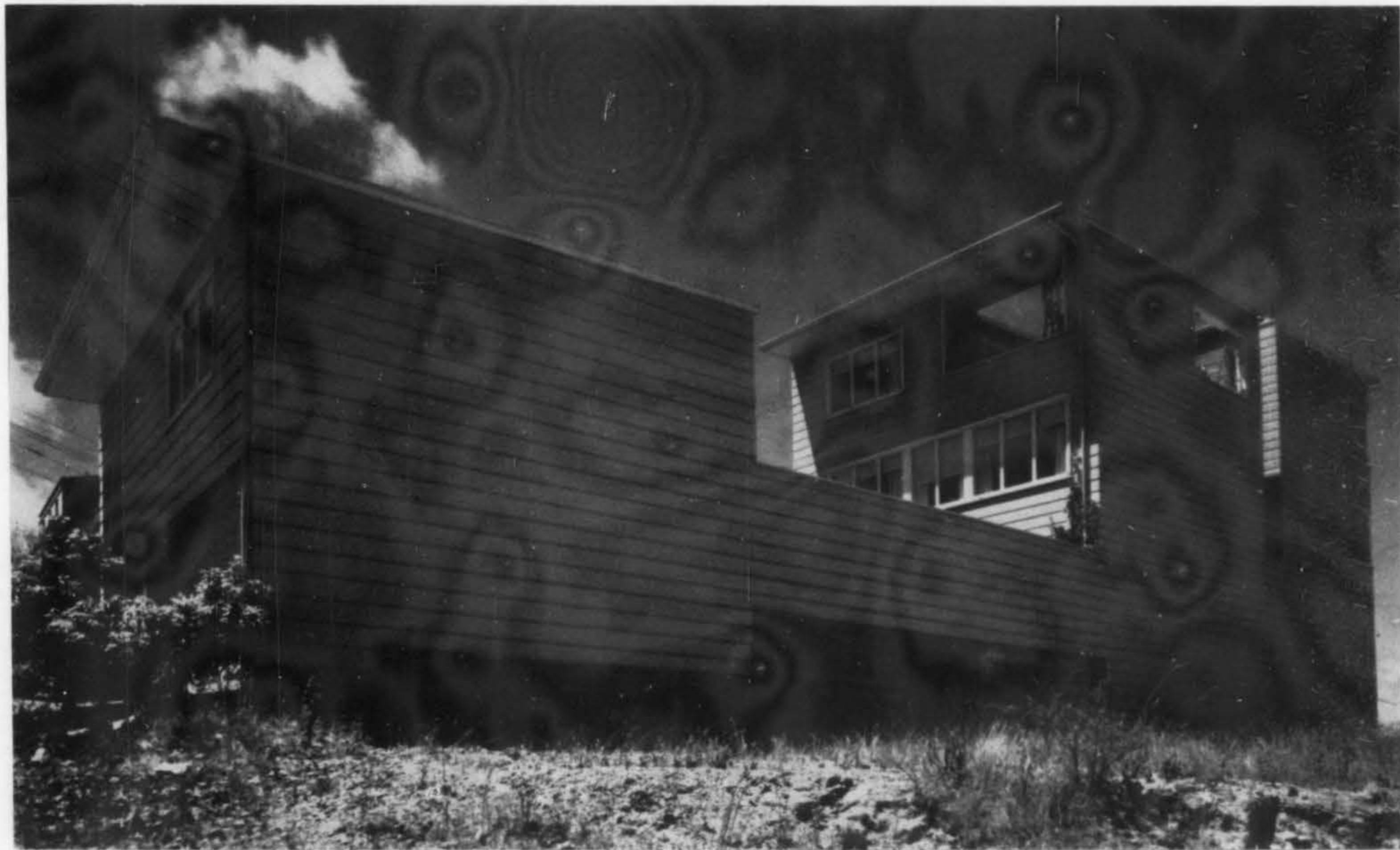
EAST VIEW OF HOUSE SHOWING SEPARATION OF GARAGE AND LIVING QUARTERS WITH OPENINGS OF THIRD FLOOR VIEW DECK. ALL EXTERIOR WALLS ARE REDWOOD SIDING
