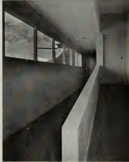
RAMPS ARE USED INSTEAD OF CONVENTIONAL STAIRWAYS
