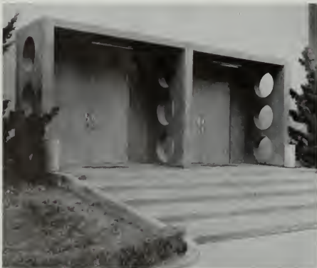
THEATER ENTRANCE SHOWING PIERCED CONCRETE FRAME
