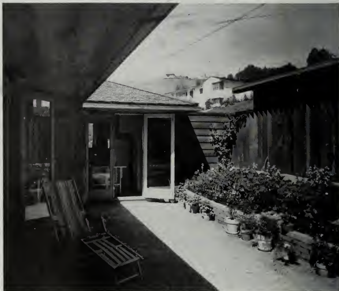
THE PRIVATE COURT SHOWING THE OVERHANG OF THE ROOF WHICH PROTECTS THE HOUSE FROM THE SUN
