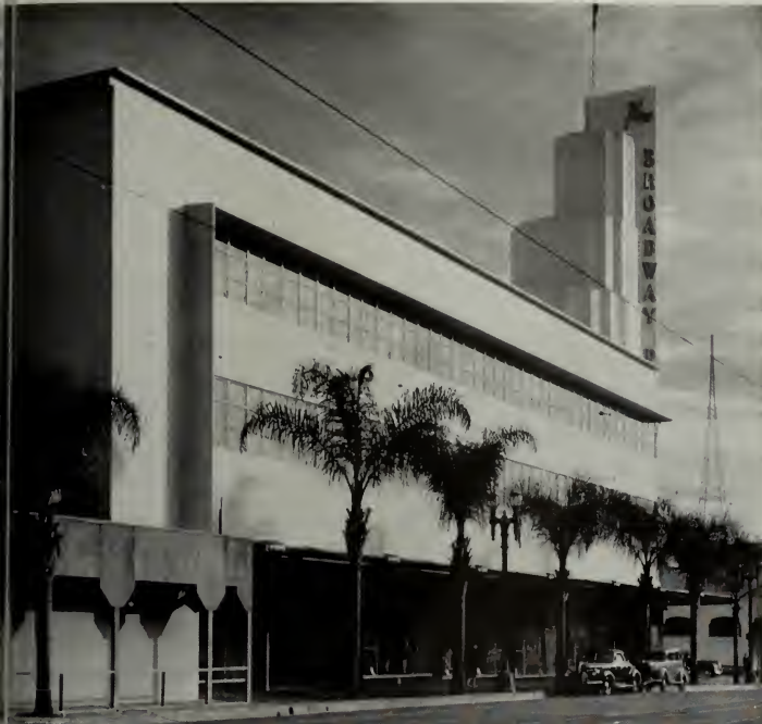
GENERAL EXTERIOR SHOWING WINDOW ARRANGEMENT, RELATION TO STREET AND USE OF SIMPLE HORIZONTAL LINES
