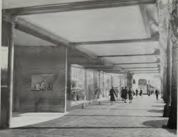
THE CANOPY EXTENDING OVER THE SIDEWALK TIED TO THE BUILDING WITH SPACED METAL STRIPS
