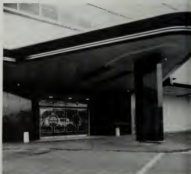
PROTECTED ENTRANCE FOR SHOPPERS DRIVEWAY
