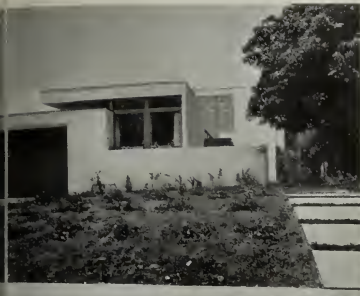
FROM THE STREET BEFORE DEVELOPMENT OF LANDSCAPING
