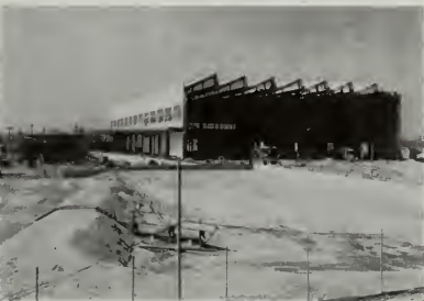
Roofs are of "saw-tooth" steel construction
