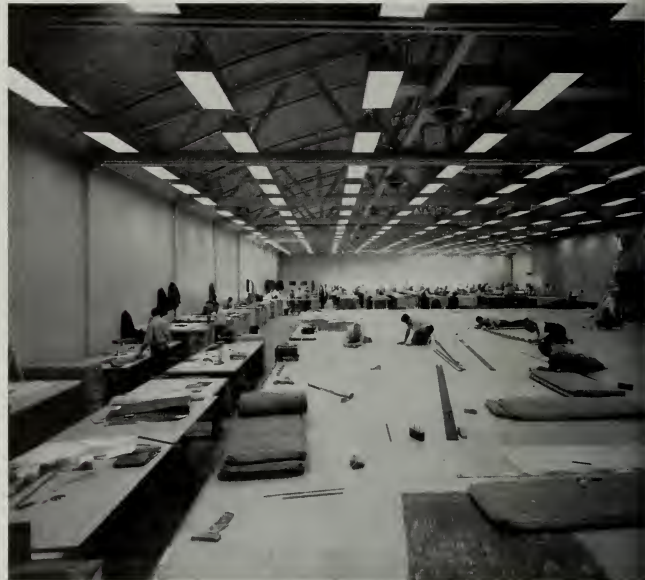
Part of the world's largest fluorescent lighting installation, used 24 hours daily. Note absence of shadows as draftsmen work on pads on drafting platform
