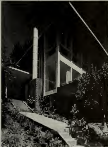
VIEW SIDE OF HOUSE SHOWING EARTHQUAKE CHIMNEY
