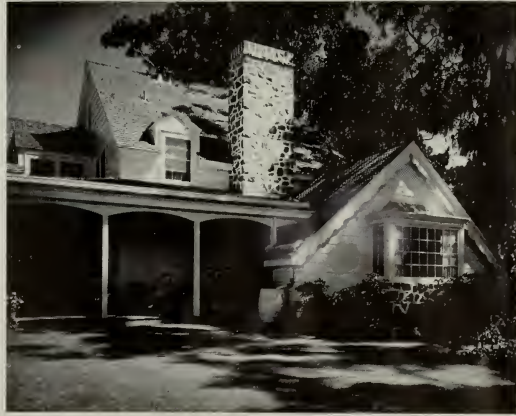
ROOF LEVELS STEP DOWN FROM THE MAIN BODY OF THE HOUSE ON THE VIEW SIDE
