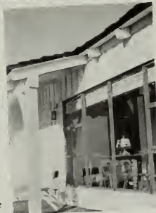
Rear terrace of the Smith home, showing vertical Redwood siding and roof shakes.
