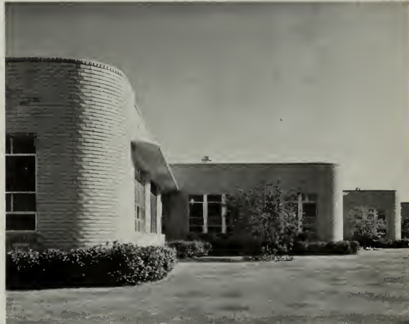
ENTRANCE TO ROTUNDA SHOWING REINFORCED GROULOCK BRICK CONSTRUCTION
