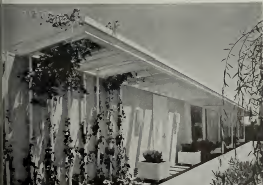
A GENEROUS OVERHANG OF THE ROOF PROTECTS THE ENTRANCE OF THE HOUSE
