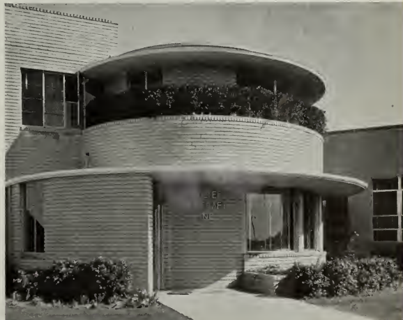
ENTRANCE TO ROTUNDA SHOWING REINFORCED GROULOCK BRICK CONSTRUCTION
